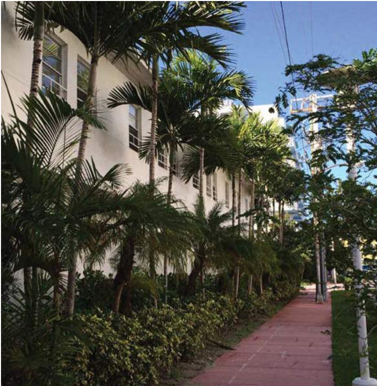
NORTH FACADE (18TH STREET)
