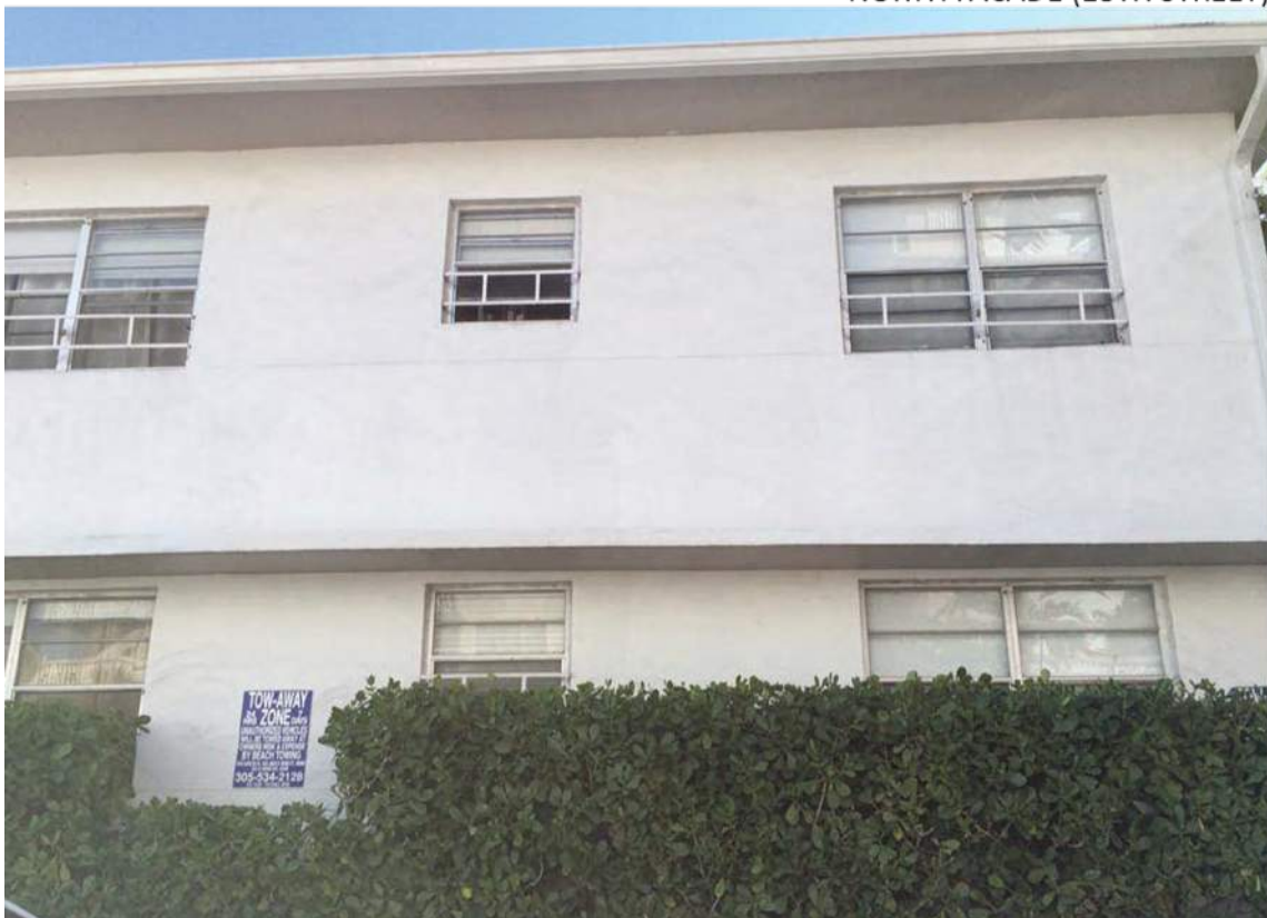
WINDOWS FACING JAMES AVENUE
