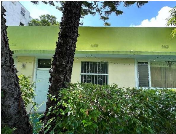
Figure 97. View of Unit 5, looking south, August 2023.
