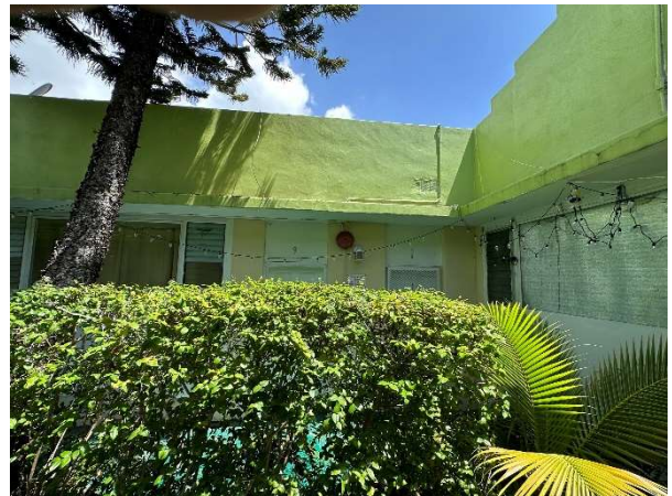
Figure 100. View of Units 8 and 9, looking northeast, August 2023.
