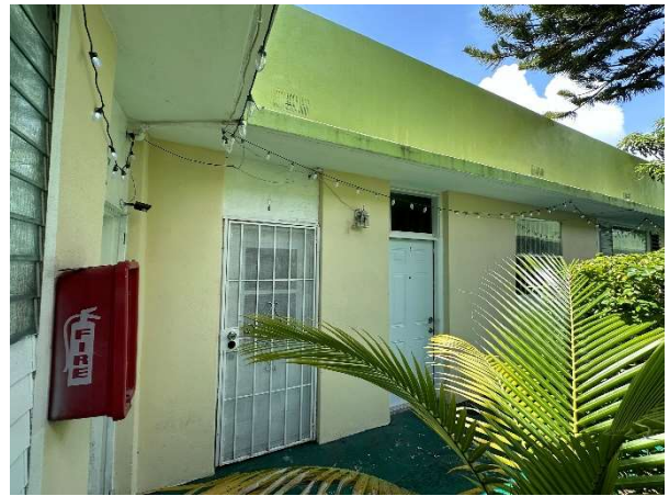
Figure 98. View of Unit 6, looking southeast, August 2023.
