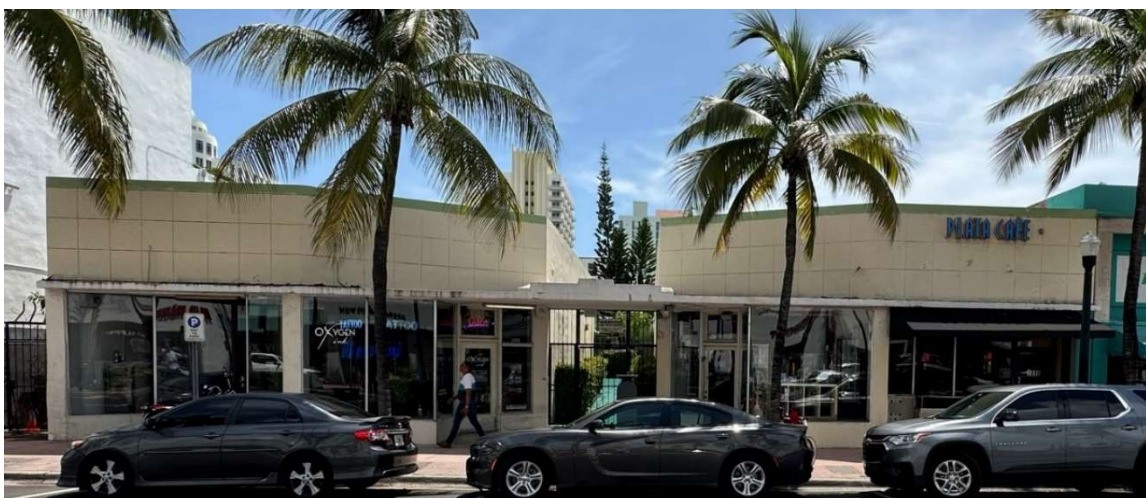
Figure 71. View of 1515-1523 Washington Avenue, looking east, August 2023.
