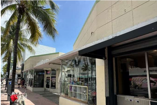
Figure 72. Detail of continuous concrete canopy, August 2023.
