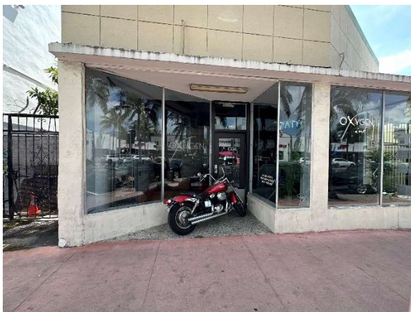
Figure 83. View of 1523 Washington Avenue, looking east, August 2023.
