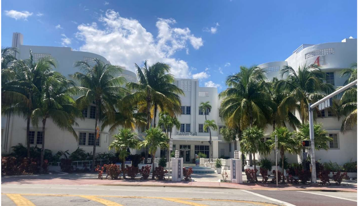
Figure 25. View of 1500 Collins Avenue, looking west, September 2023.
