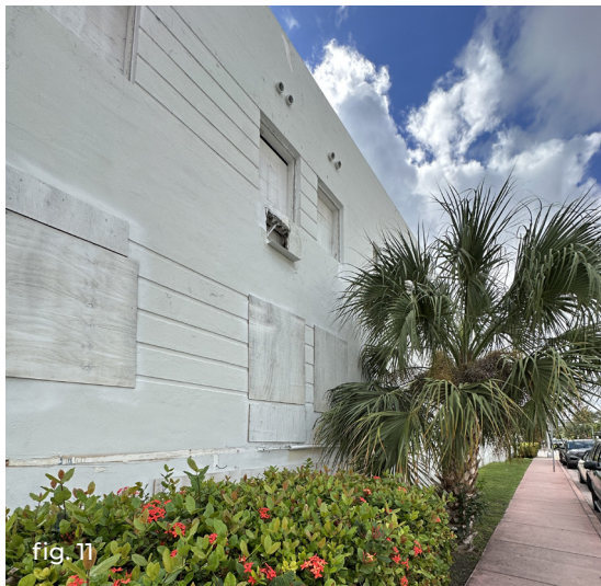
North Facade | Board-up Windows | March 2024
