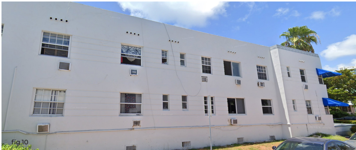
East Facade | WALL UNIT AC | July 2018
