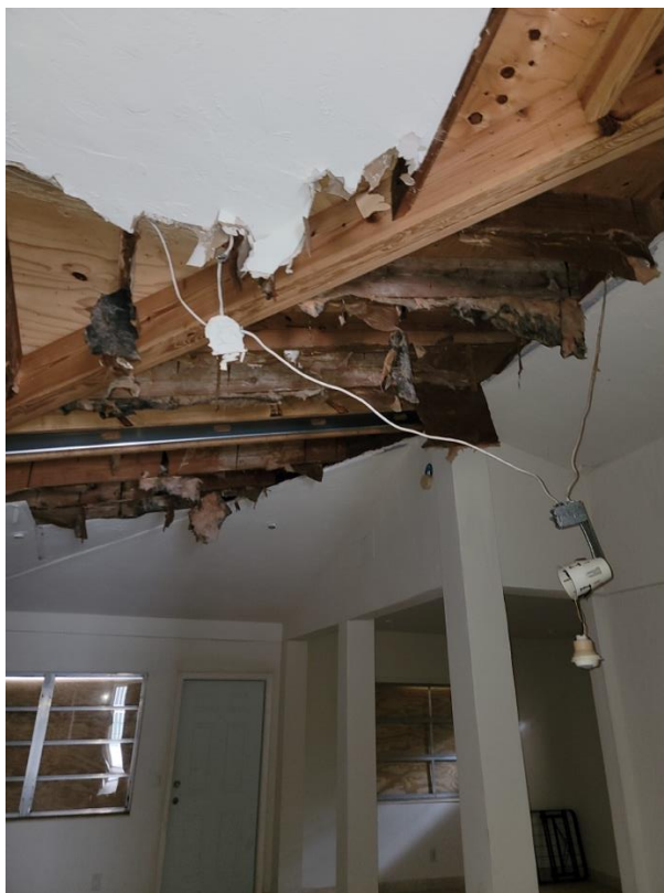
Water intrusion from the roof lead to damage of roof decking, and roof joists
