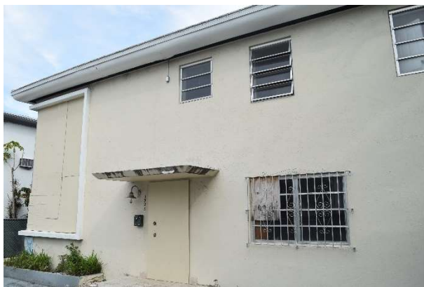
Figure 48. View of west elevation, looking northeast, February 2024.
