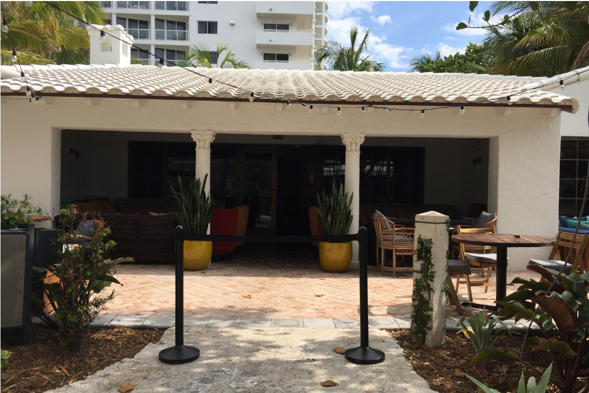
VIEW 5: NOUTH ENTRANCE FROM POOL
