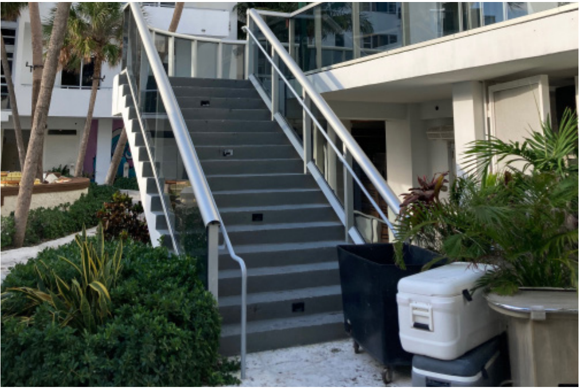
VIEW 2: SECOND FLOOR ACCESS
