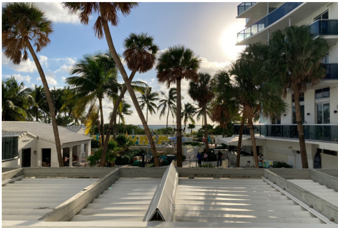
VIEW 9: SECOND FLOOR CORRIDOR VIEW
