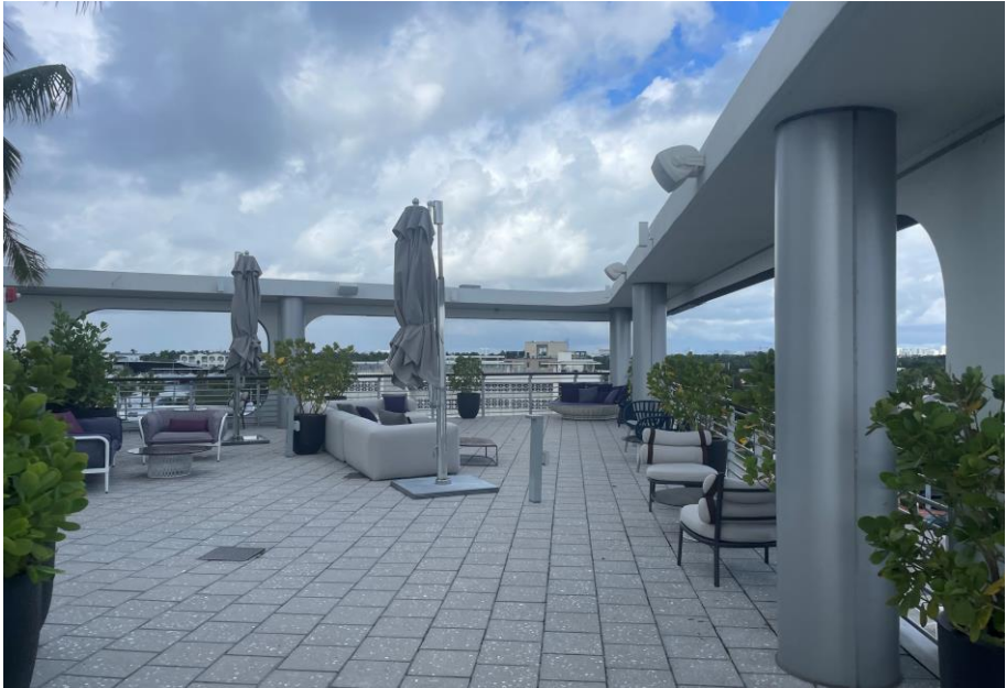
3 ROOF TERRACE / NORTH
