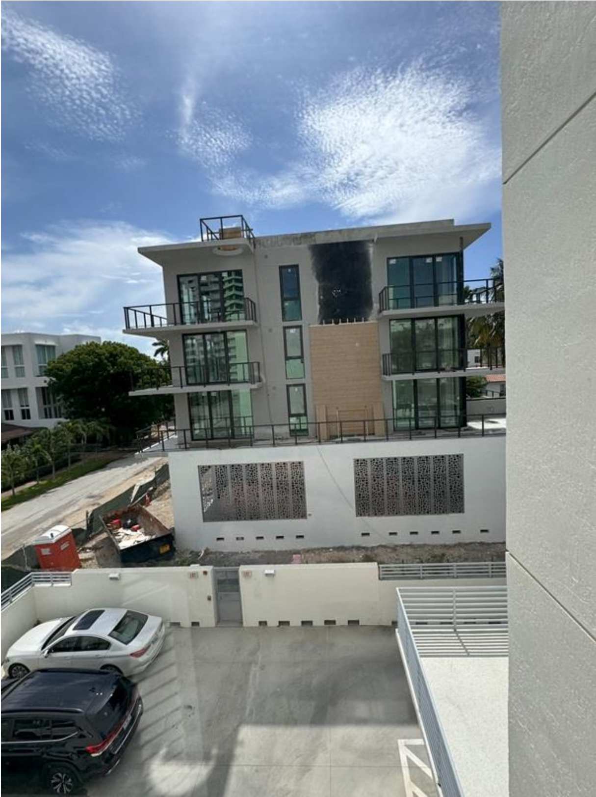
1414 West Ave construction blocking view from one bedroom already
