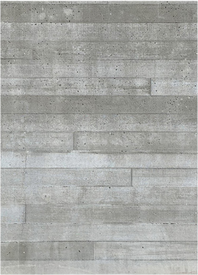
7. ARCHITECTURAL FEATURE WALL BOARD FORMED CONCRETE
