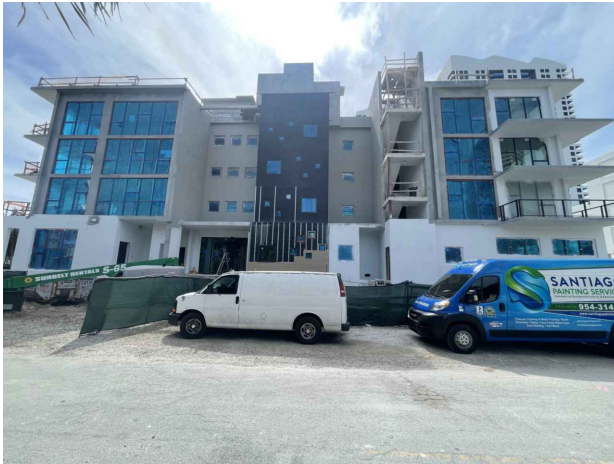
EAST NEIGHBOR CONSTRUCTION (8)
