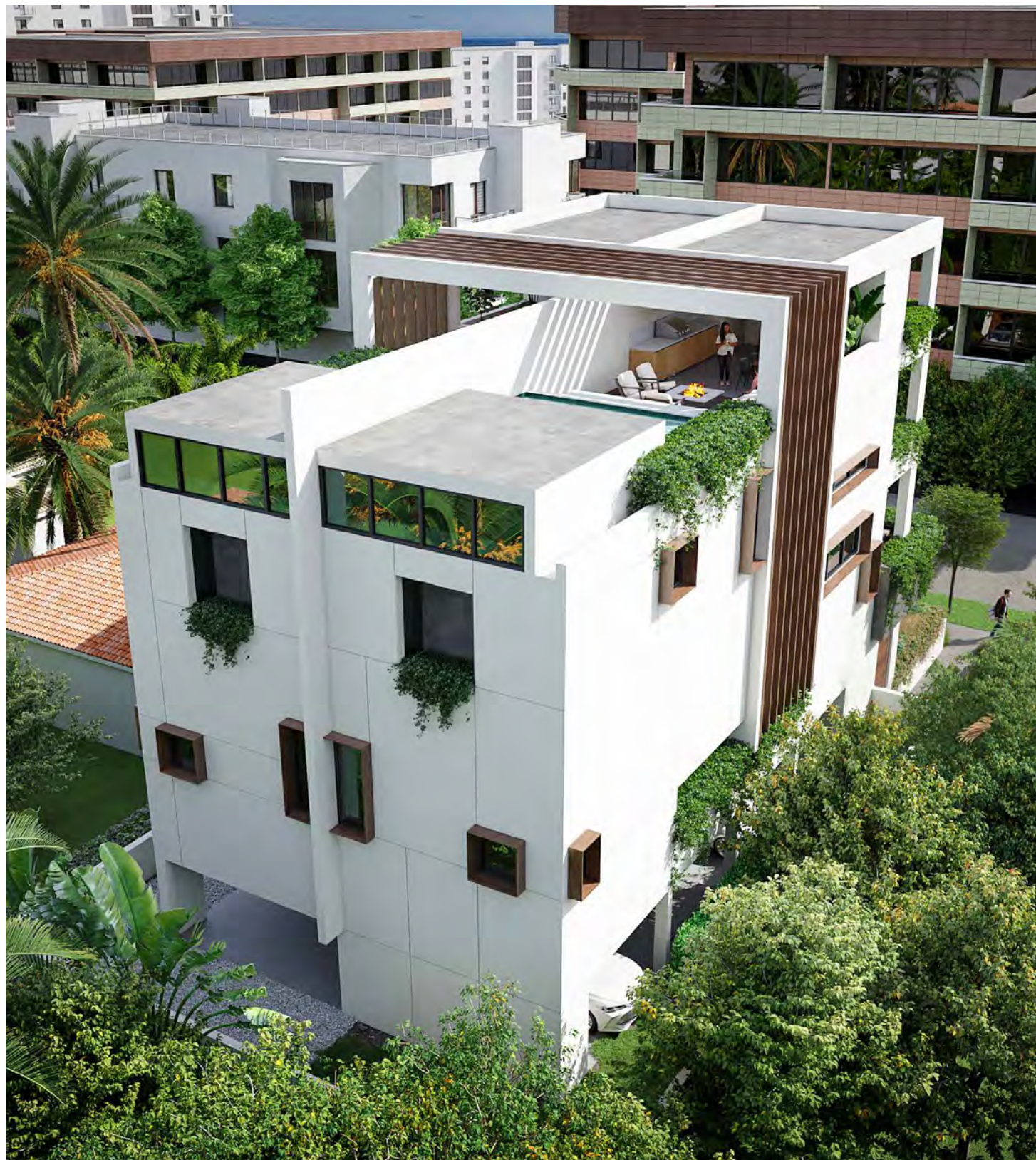
REAR VIEW FROM NORTH WEST
