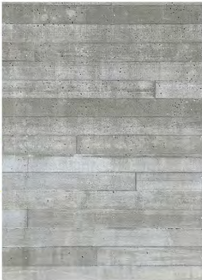
7. ARCHITECTURAL FEATURE WALL BOARD FORMED CONCRETE
