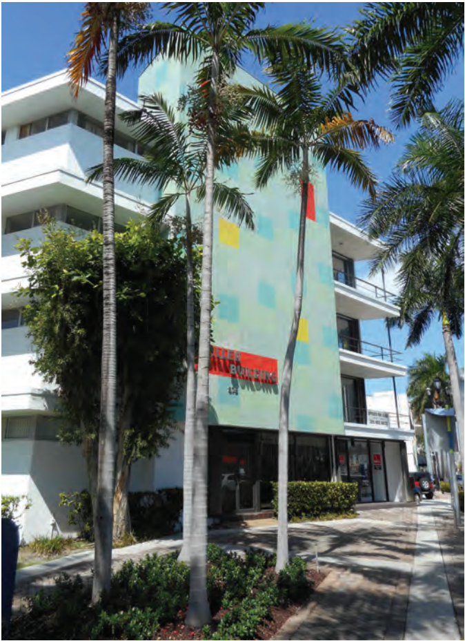
NORTH@ 41 ST. - GILLER BUILDING
