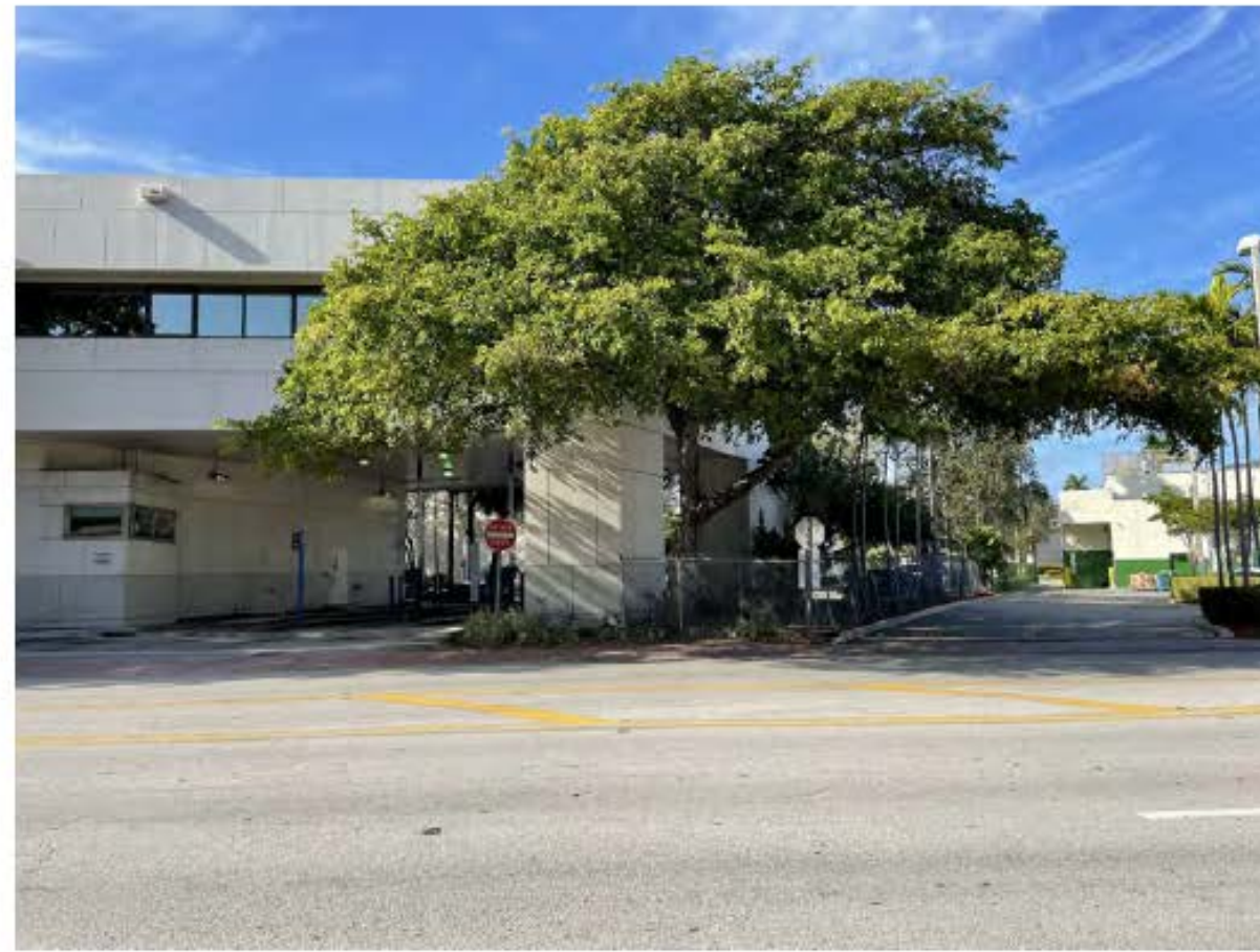
06 DADE BOULEVARD LOOKING NORTH
