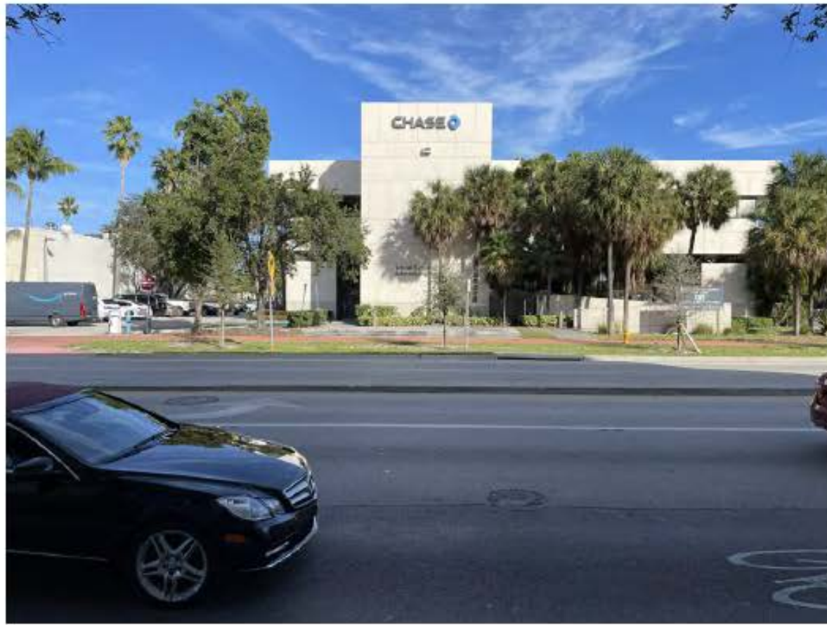
01 ALTON ROAD LOOKING EAST AT 1801 ALTON ROAD
