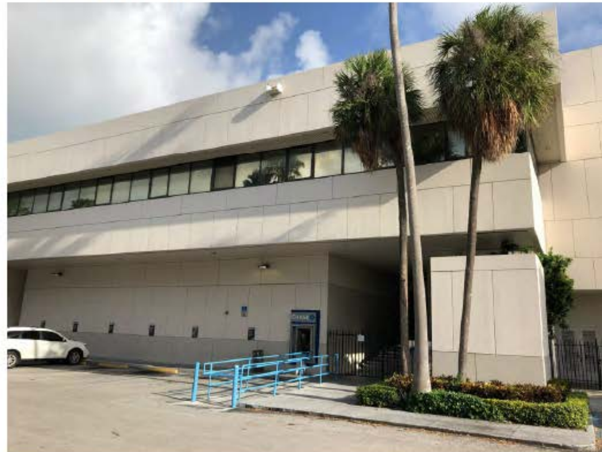
08 EXISTING PARKING LOT LOOKING SOUTH
