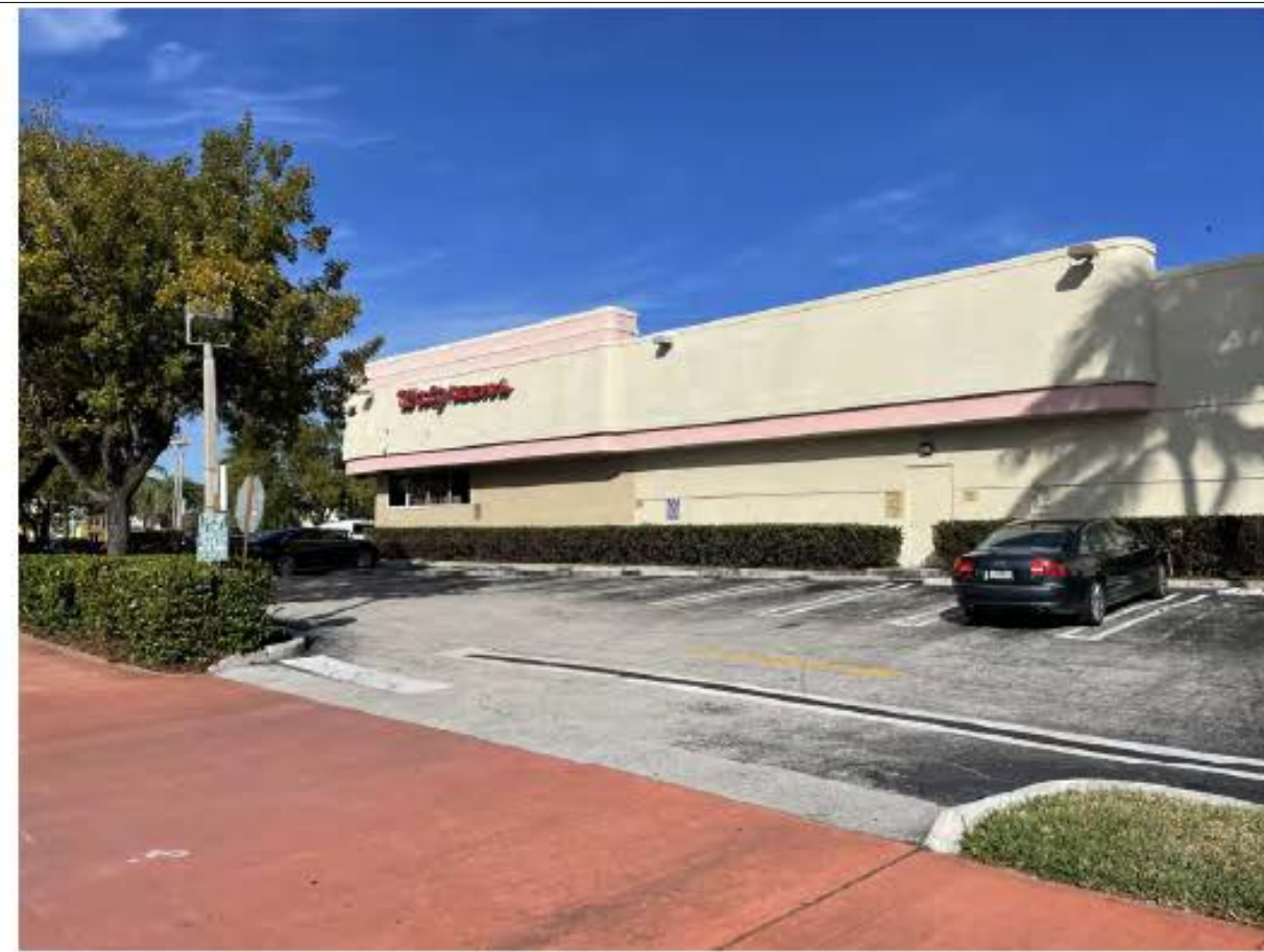
22 ALTON ROAD LOOKING NORTH EAST AT WALGREENS
