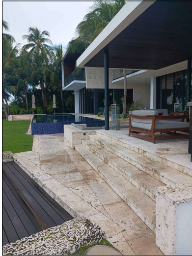
① REAR LOOKING NORTHWEST
