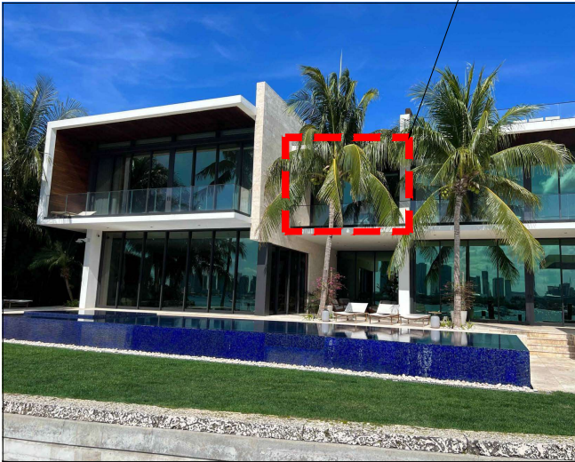
① REAR - LOOKING NORTH EXISTING
