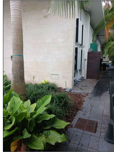
② SIDE LOOKING SOUTHEAST
