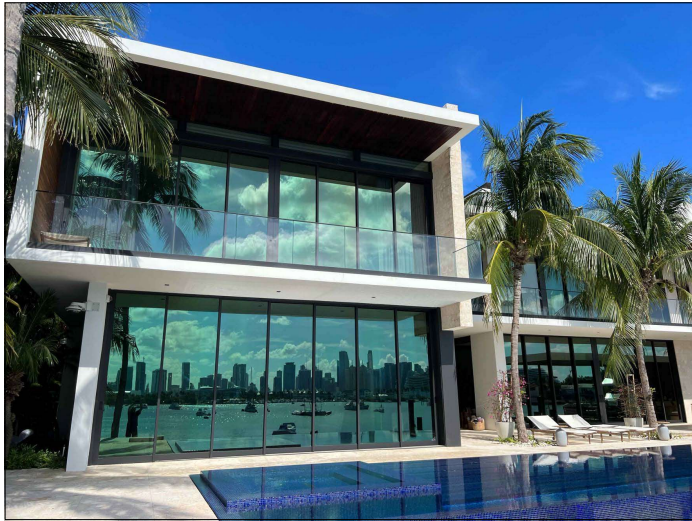
③ REAR LOOKING NORTH
