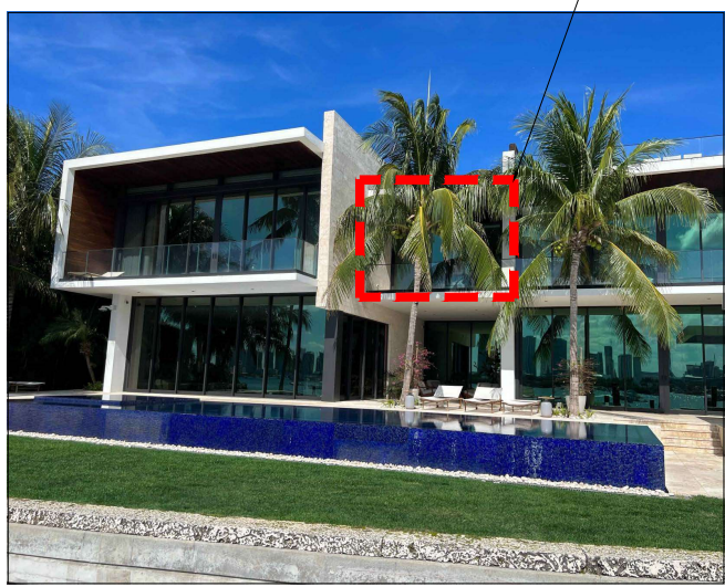
① REAR - LOOKING NORTH EXISTING
