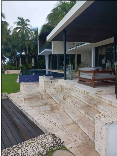
① REAR LOOKING NORTHWEST
