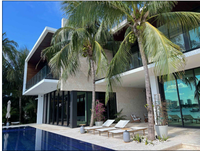
④ REAR - LOOKING NORTHWEST
