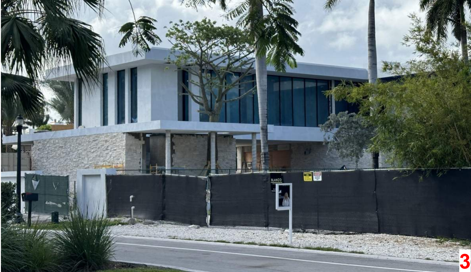
111 PALM AVE - UNDER CONSTRUCTION
