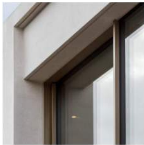
GL-01 IMPACT GLAZING - CLEAR W/ BRONZE FRAME
