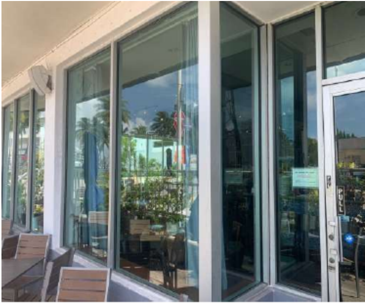
ORIGINAL 18TH ST FACADE
