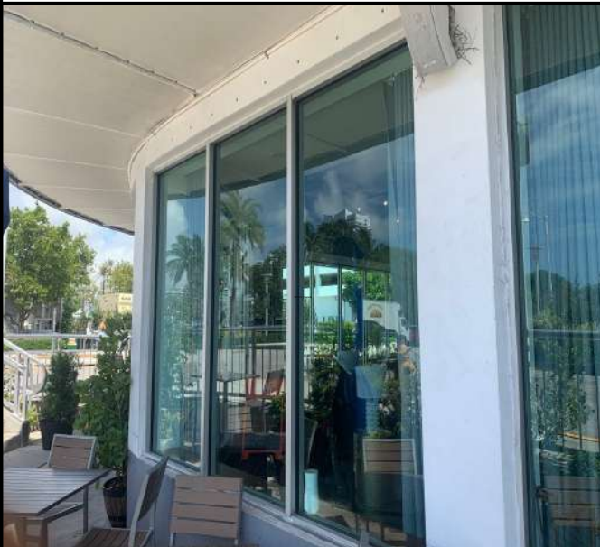
ORIGINAL 18TH ST FACADE
