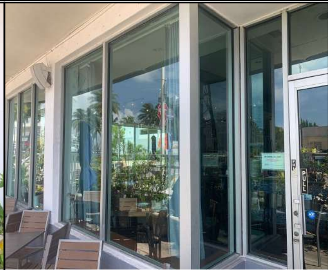
ORIGINAL 18TH ST FACADE
