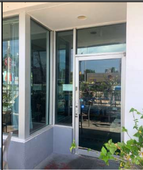
ORIGINAL 18TH ST FACADE
