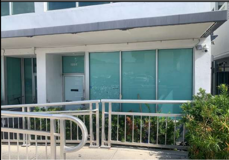
ORIGINAL 18TH ST FACADE
