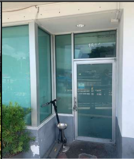
ORIGINAL 18TH ST FACADE
