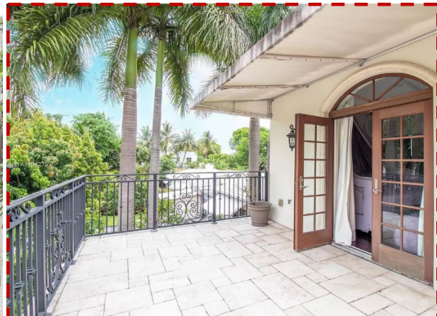
Roof balcony to be enclosed.
