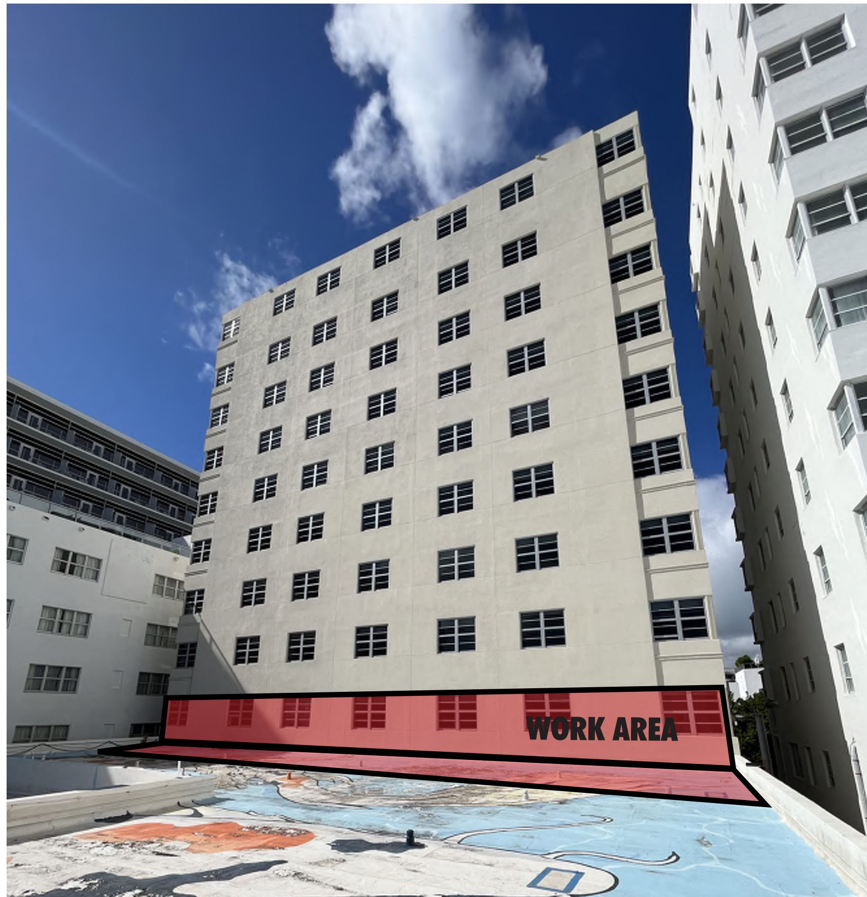
PHOTO AT 3RD FL. ROOF LEVEL
