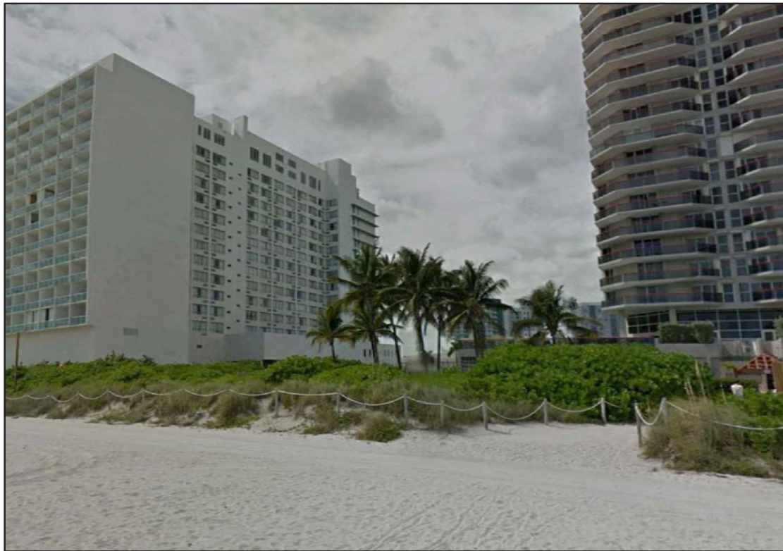
C - NORTHEAST VIEW OF THE SITE
