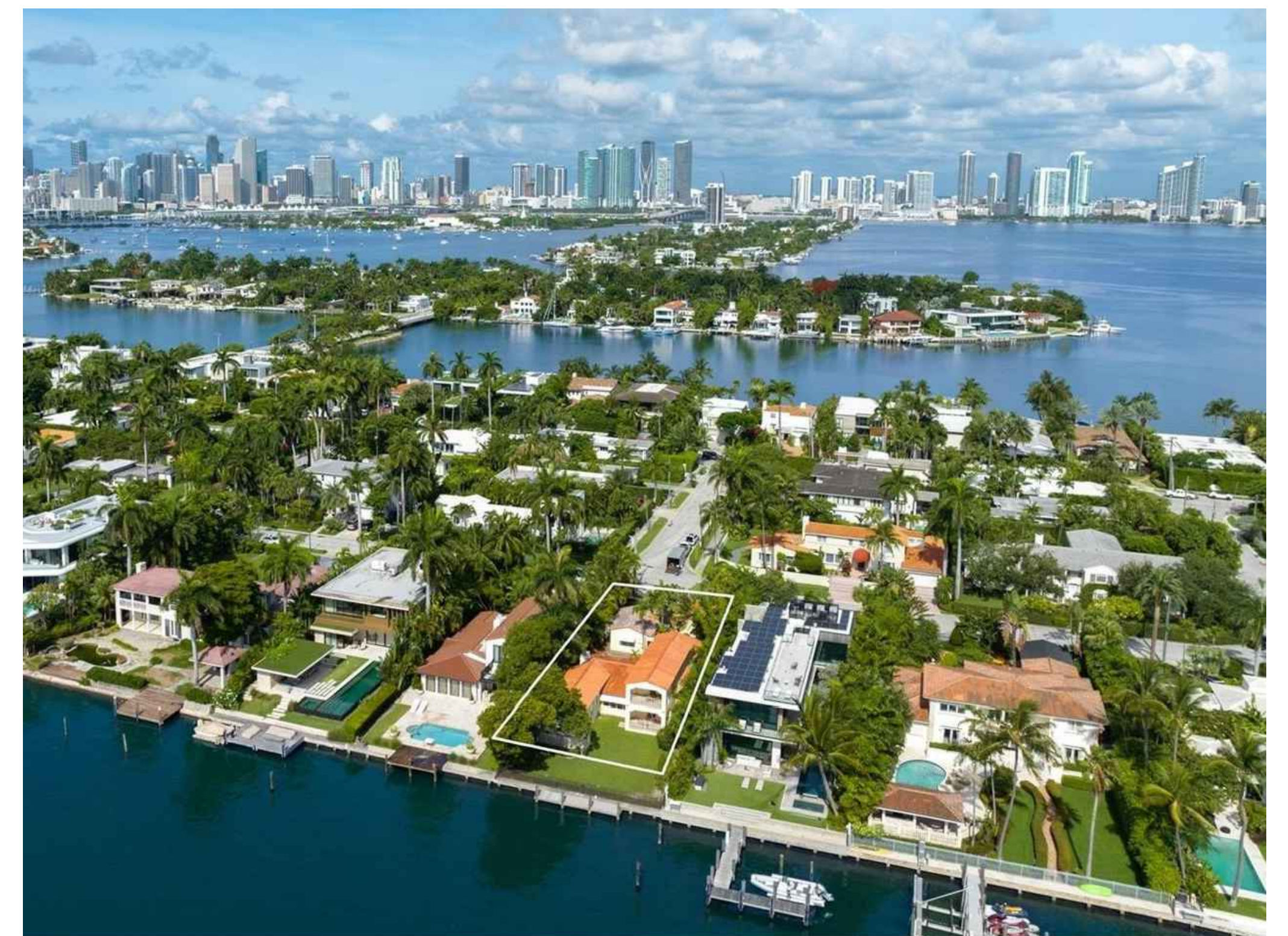
A3 AERIAL PHOTO - VIEW TO THE REAR OF THE PROPERTY
