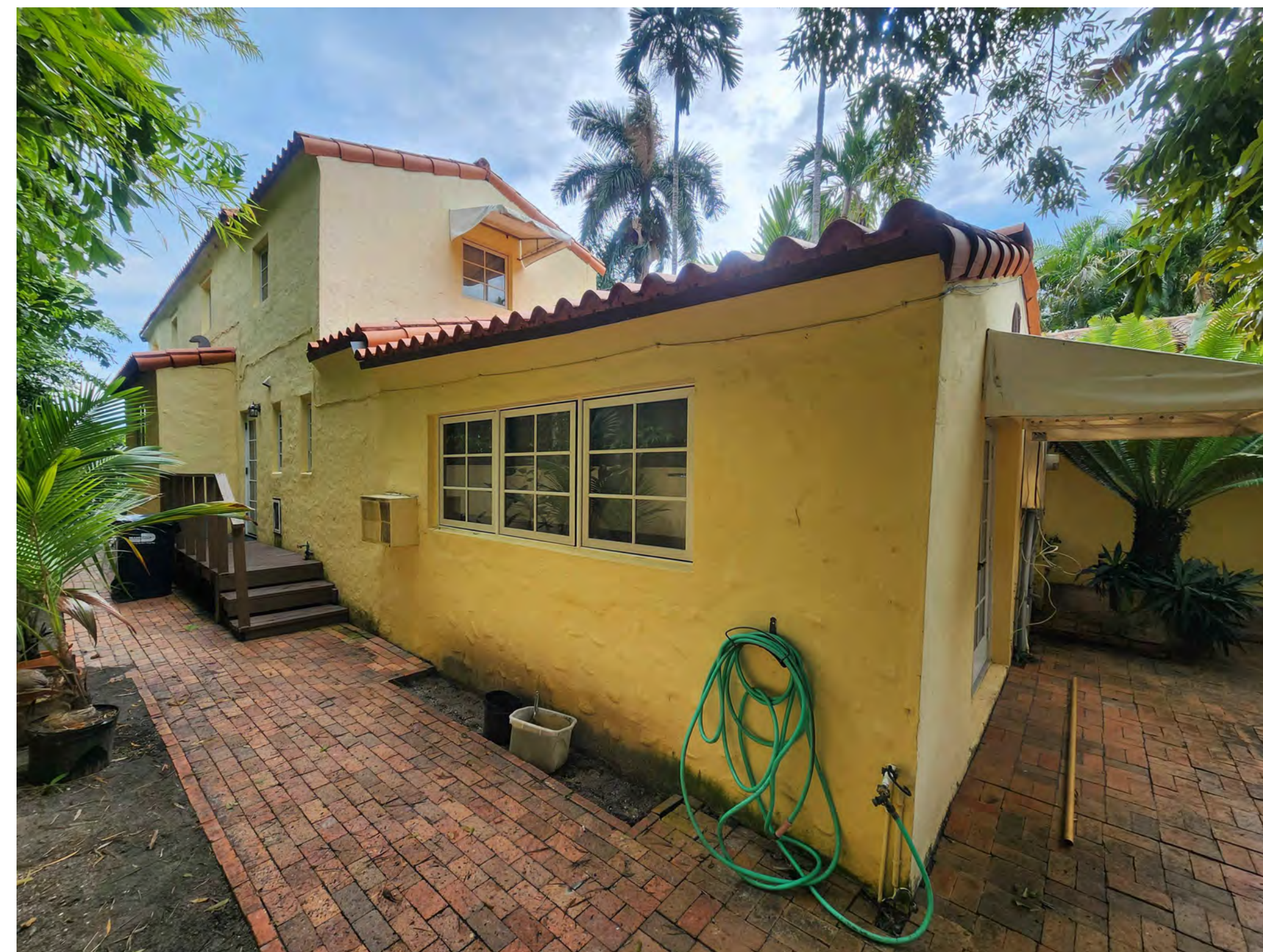
A2 NORTH SIDE VIEW PATIO SHOWING: THE 1935 ORIGINALLY BUILT MAIN HOUSE, INCLUDING THE ADDITION AND GARAGE CONVERSION INTO A BEDROOM IN 1955 AND 2007 ADDITION TO KITCHEN SPACE (PHOTO TAKEN: 12/23/2022)
