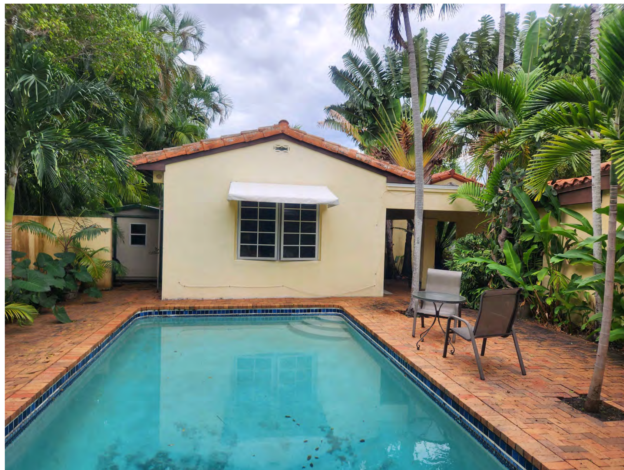
A1 INTERIOR PATIO VIEW SHOWING: THE GUEST HOUSE WAS ORIGINALLY BUILT IN 1955 AND GALLERY (PHOTO TAKEN: 12/23/2022)
