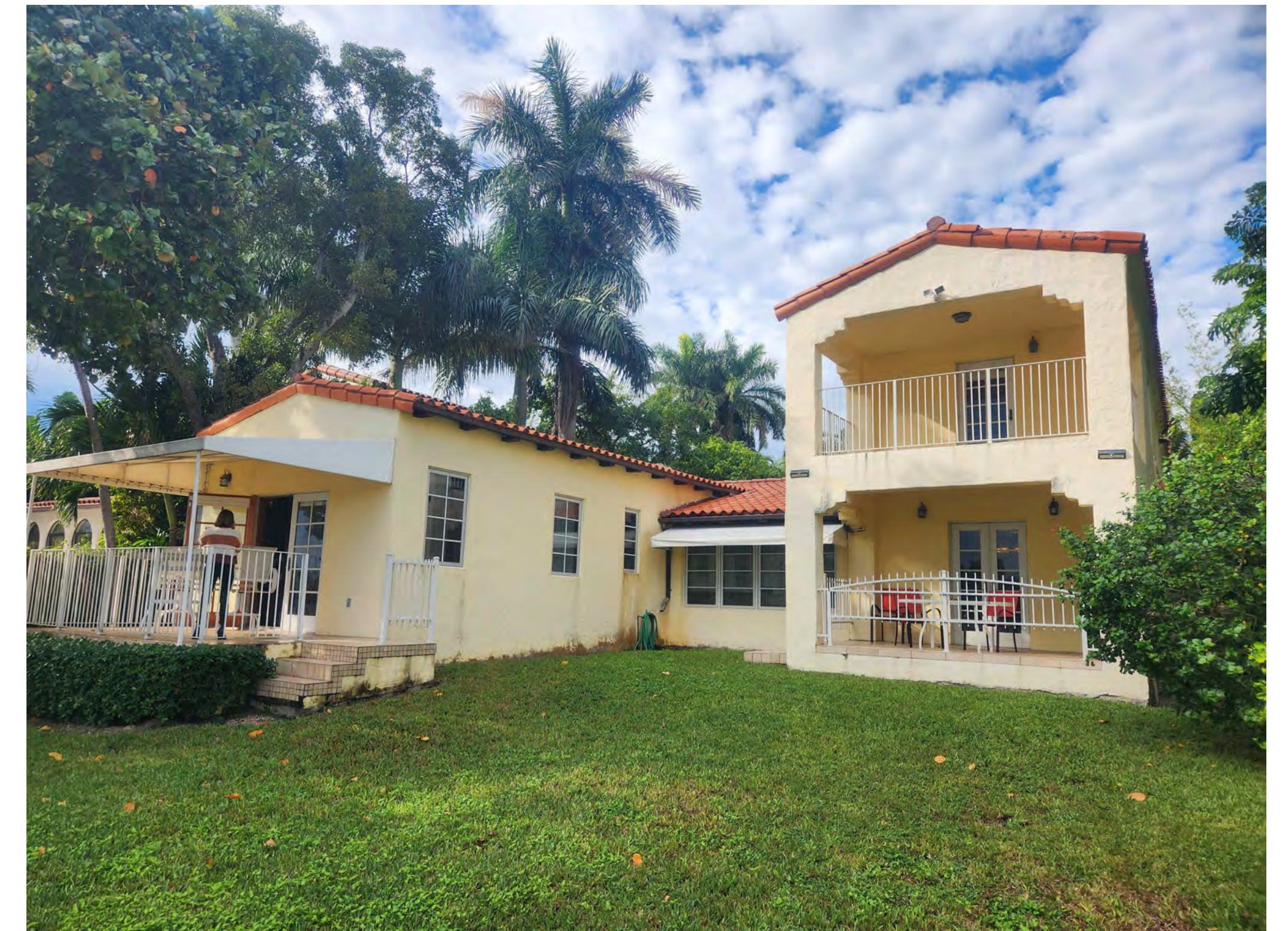
B3 MAIN HOUSE REAR VIEW IMAGE SHOWING: THE NEW ADDITIONS BUILT IN 2007, THE MASTER SUITE TO THE LEFT SIDE AND TWO STORY COVERED TERRACE AND BALCONY AT SECOND FLOOR (PHOTO TAKEN: 12/23/2022)
