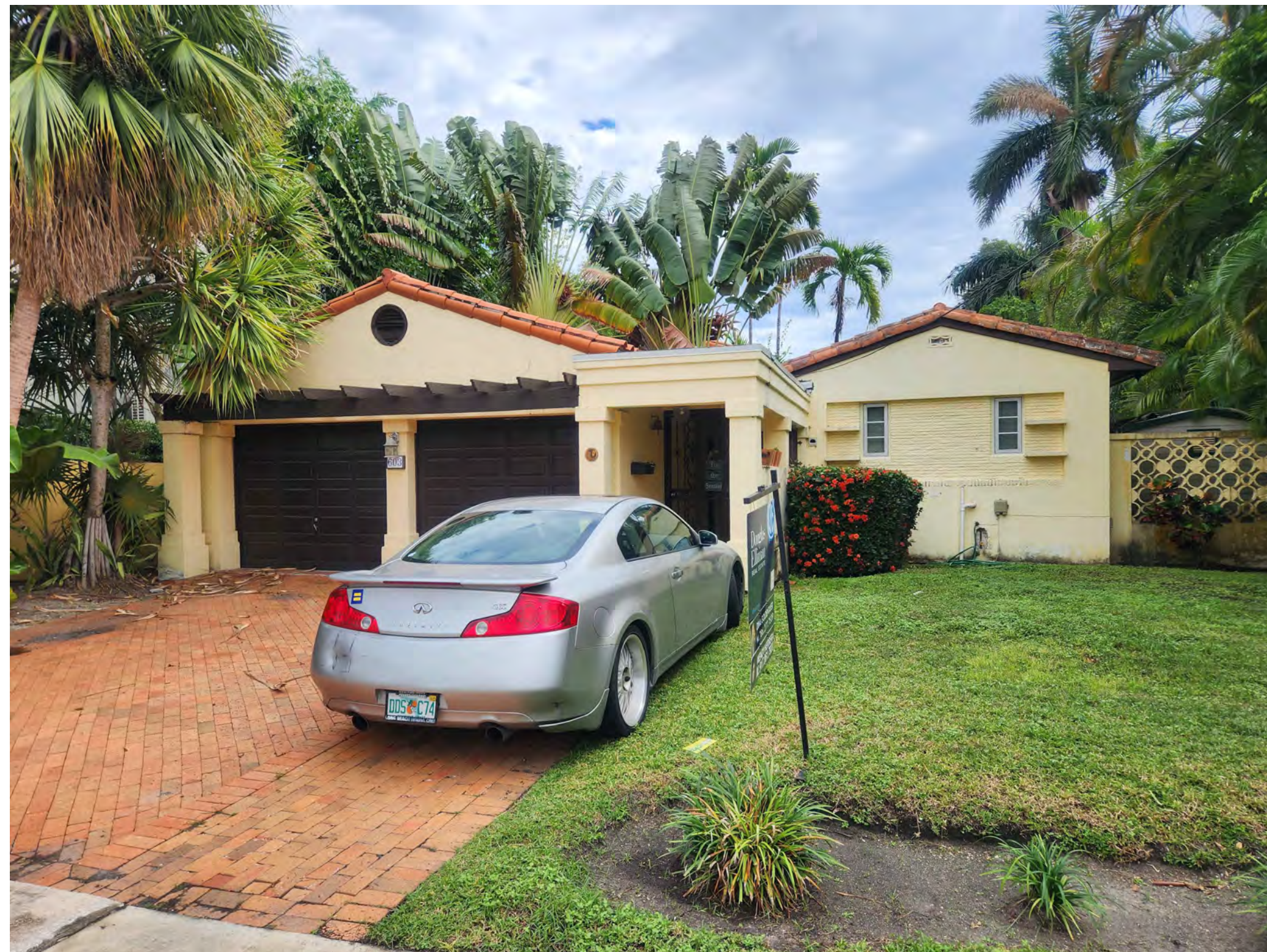
B1 VIEW FROM THE STREET SHOWING: THE GUEST HOUSE, ORIGINALLY BUILT IN 1955, INCLUDING THE COVERED ENTRY GALLERY. THE DETACHED GARAGE WAS BUILT IN 1990 (PHOTO TAKEN: 12/23/2022)
