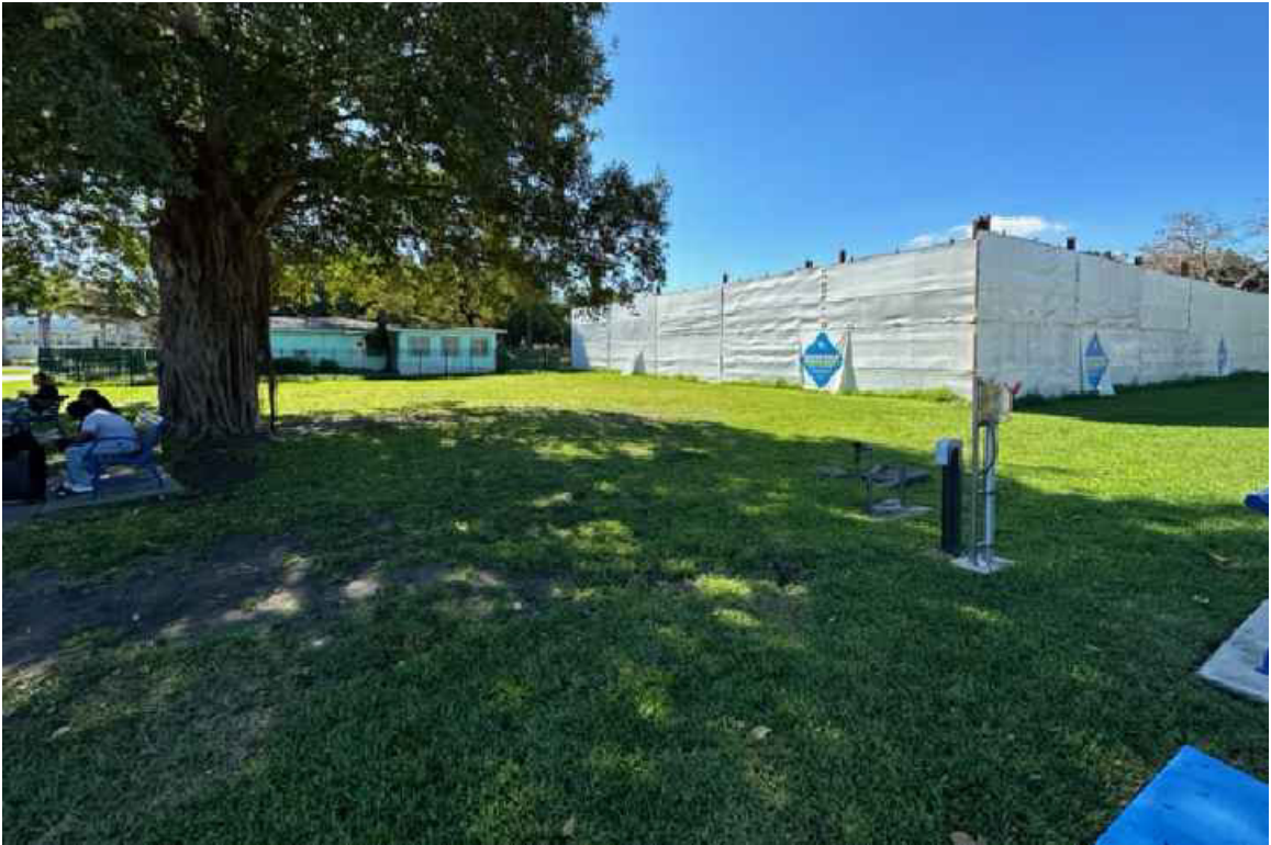
8. LODGING AND FPL STAGING AREA
