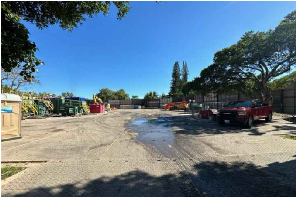
13. INSIDE FPL STAGING AREA
