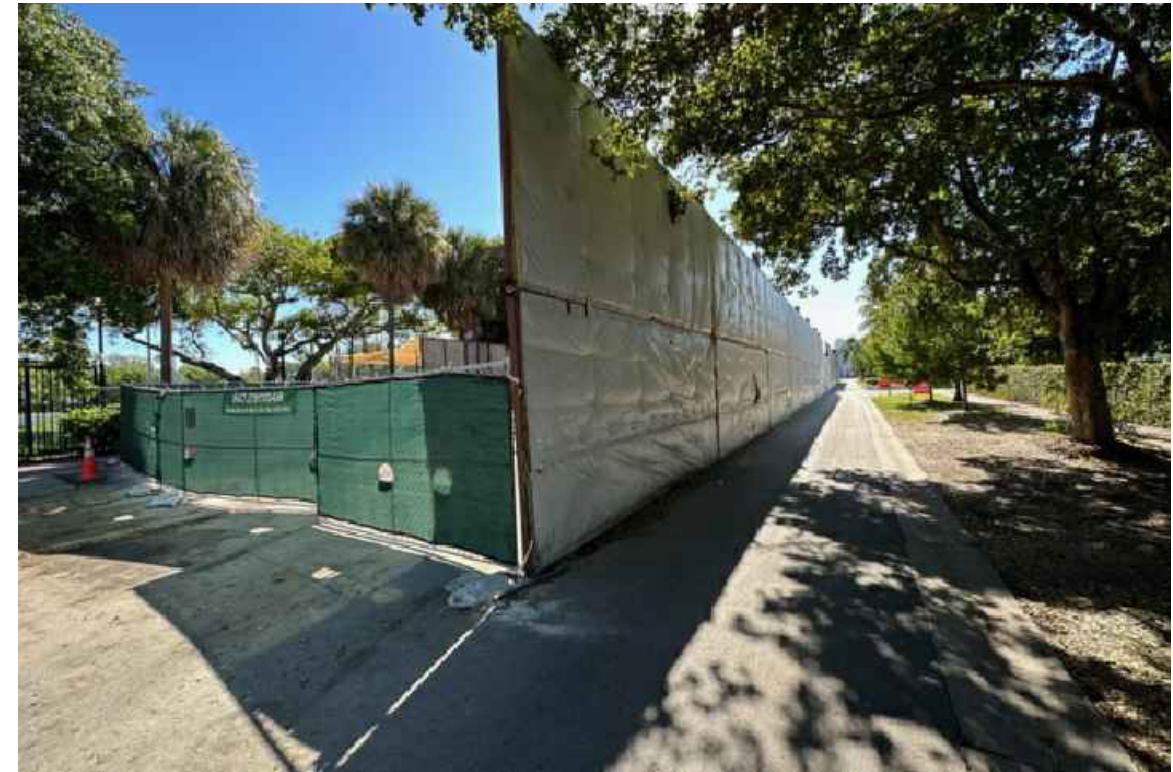
6. FPL WORK ON MICHIGAN AVENUE
