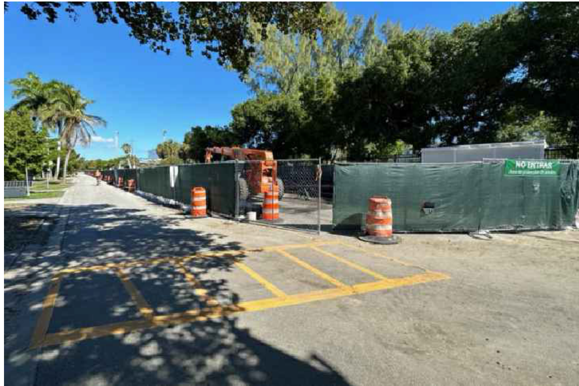
5. FPL WORK ON MICHIGAN AVENUE
