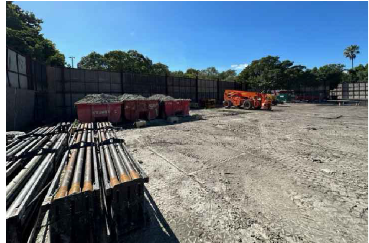
16. INSIDE FPL STAGING AREA FACING MICHIGAN AVENUE
