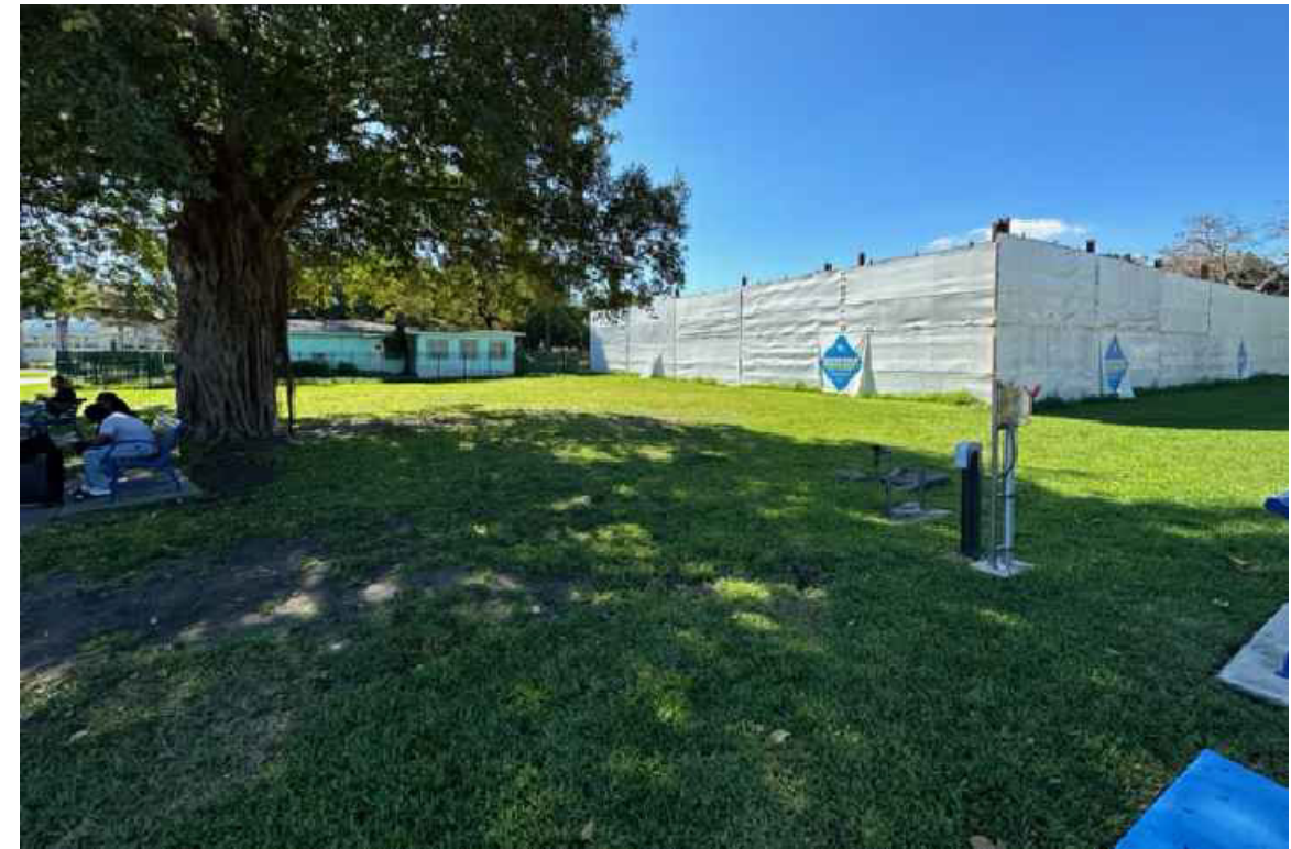
8. LODGING AND FPL STAGING AREA
