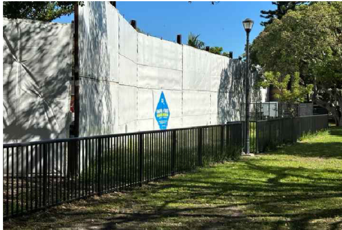
11. FENCE BETWEEN PLAYGROUND AND FPL STAGING AREA, ELECTRICAL PANEL AND METER TOWARDS THE BACK
