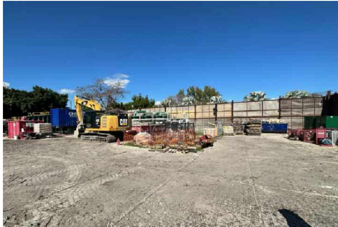
17. INSIDE FPL STAGING AREA LOOKING AT MICHIGAN AVENUE
