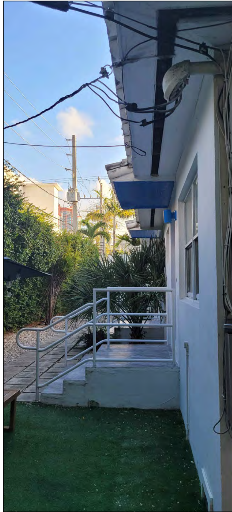
STAIRS STOOPS AND RAILINGS TO BE DEMOLISHED
