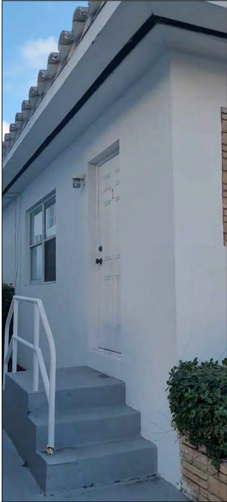
STAIRS STOOPS AND RAILINGS TO BE DEMOLISHED
