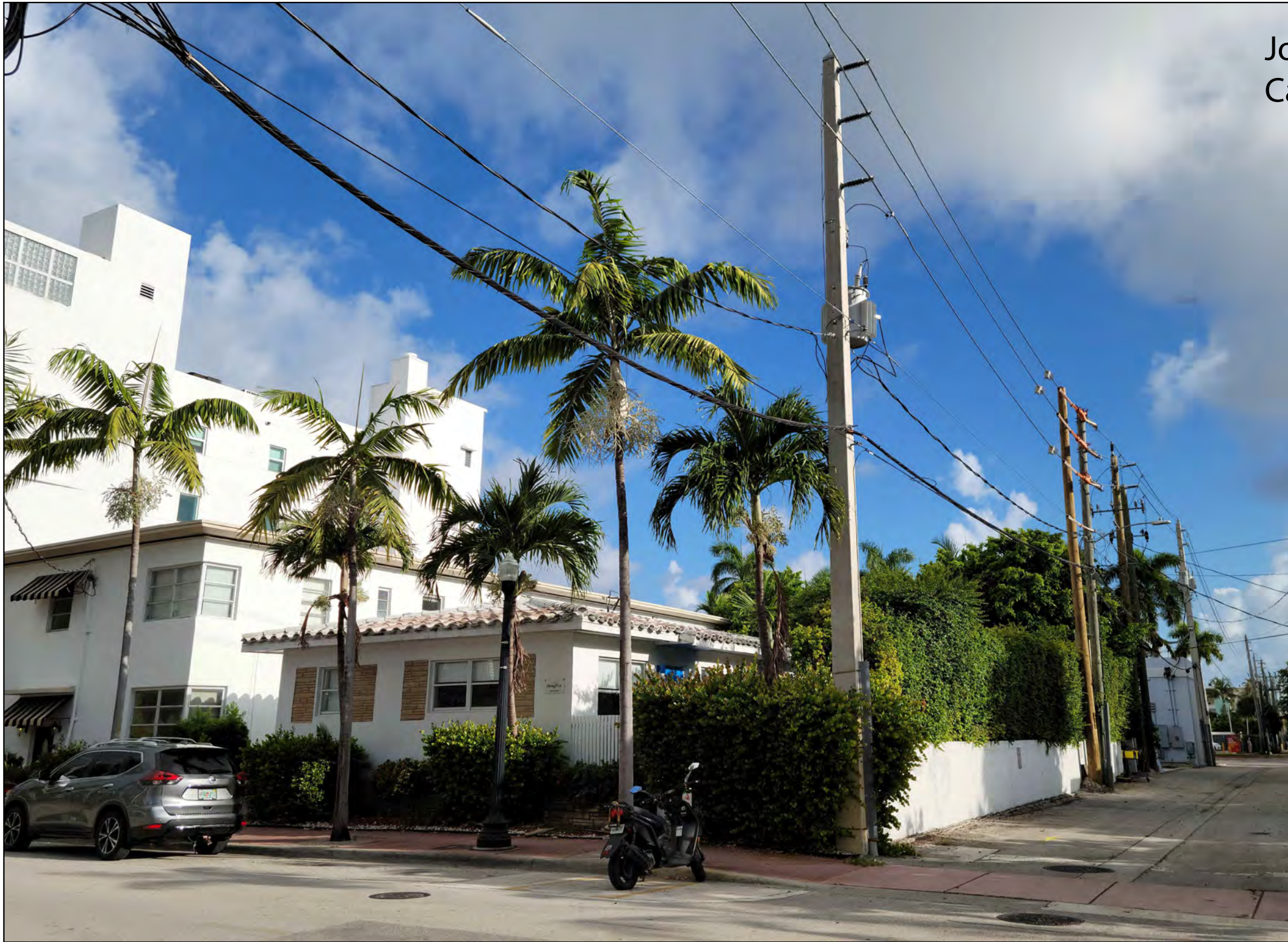
16. STREET FACADE VIEW @ 4TH 5 AND ALLEY
