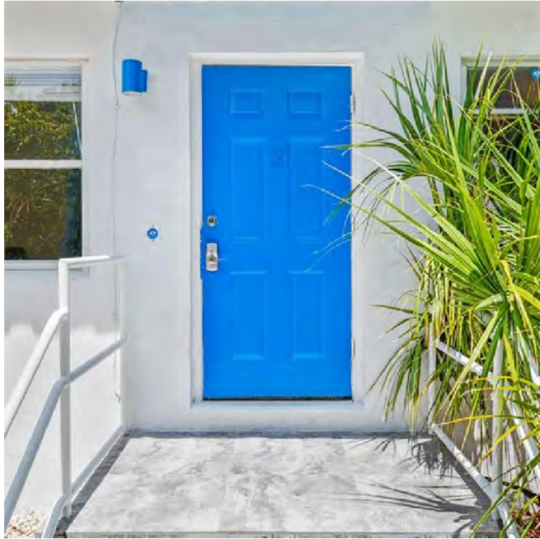
TYPICAL ENTRY DOOR
