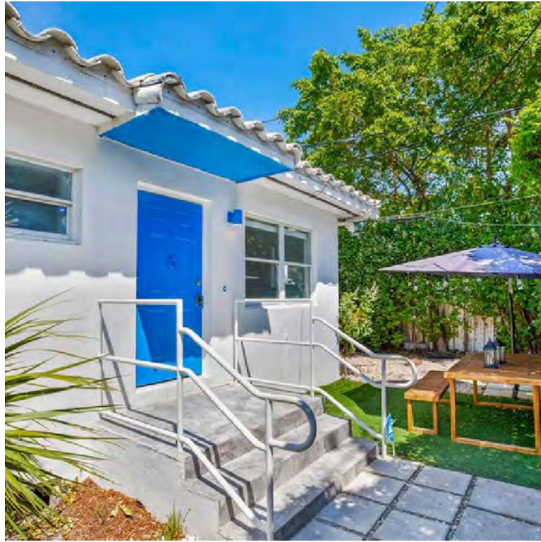
STAIR STOOP AND HANDRAILS
