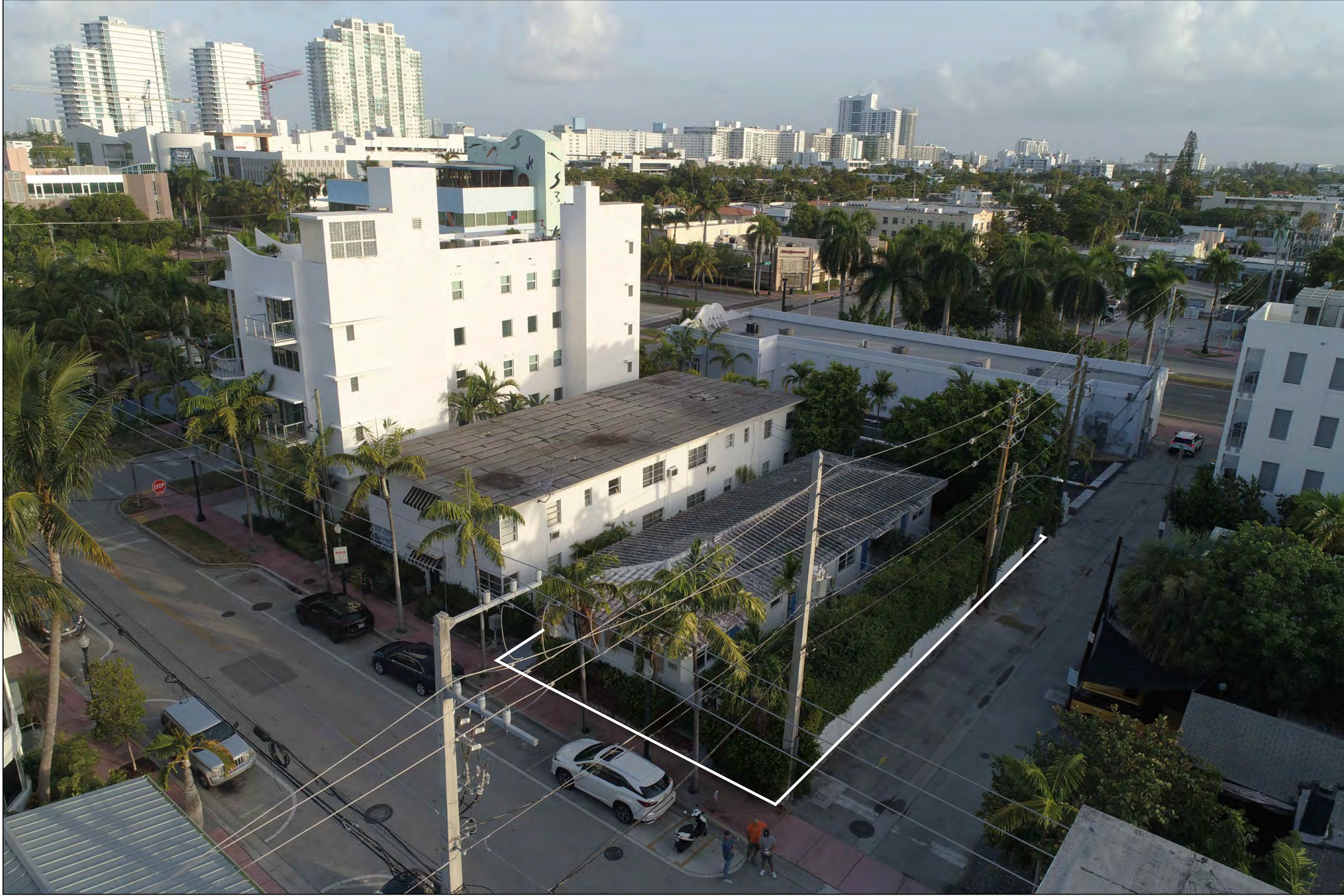
6. AERIAL VIEW OF 829 4TH STREET FACING NW
