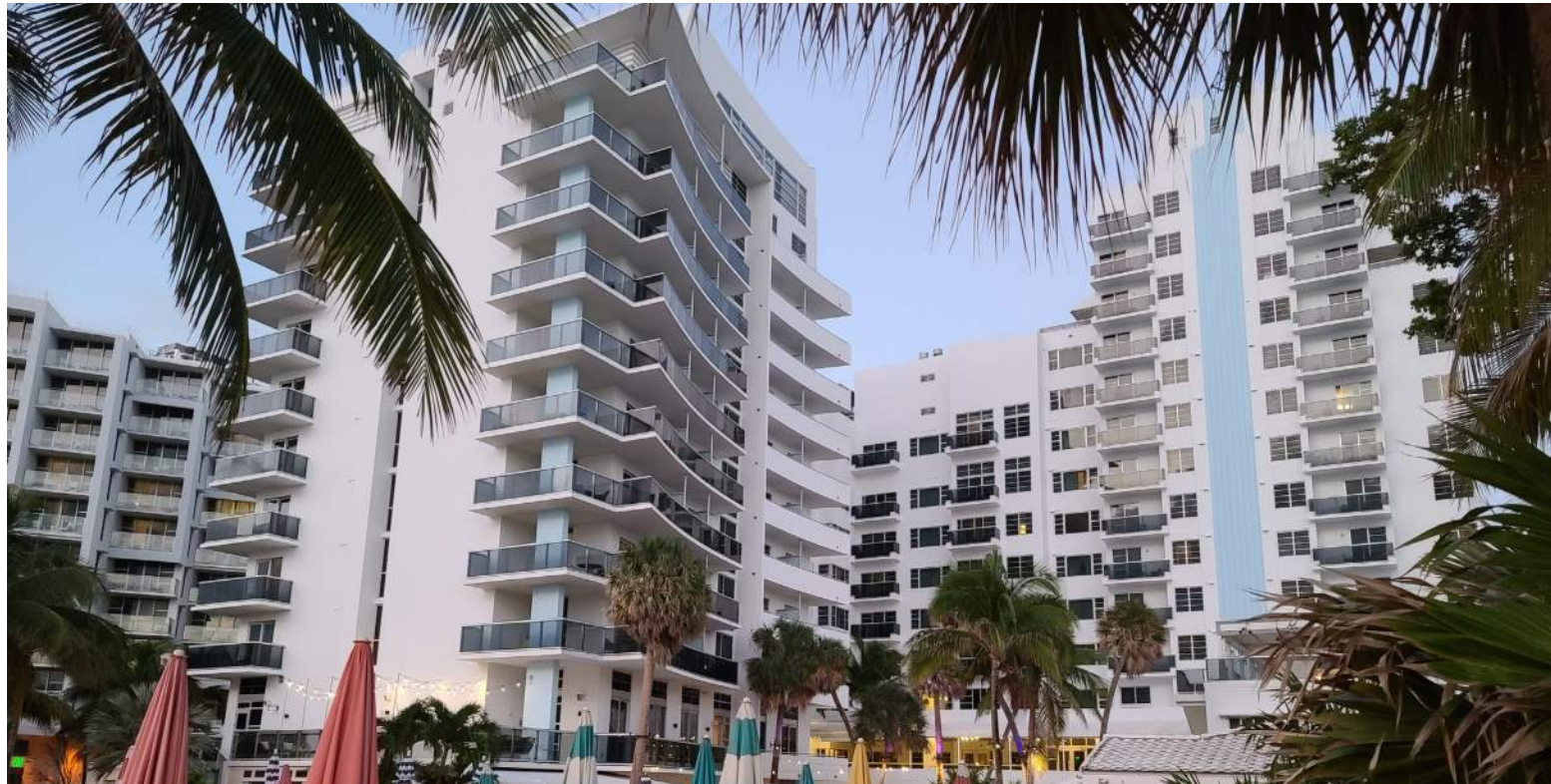
NORTH EAST FACADE
