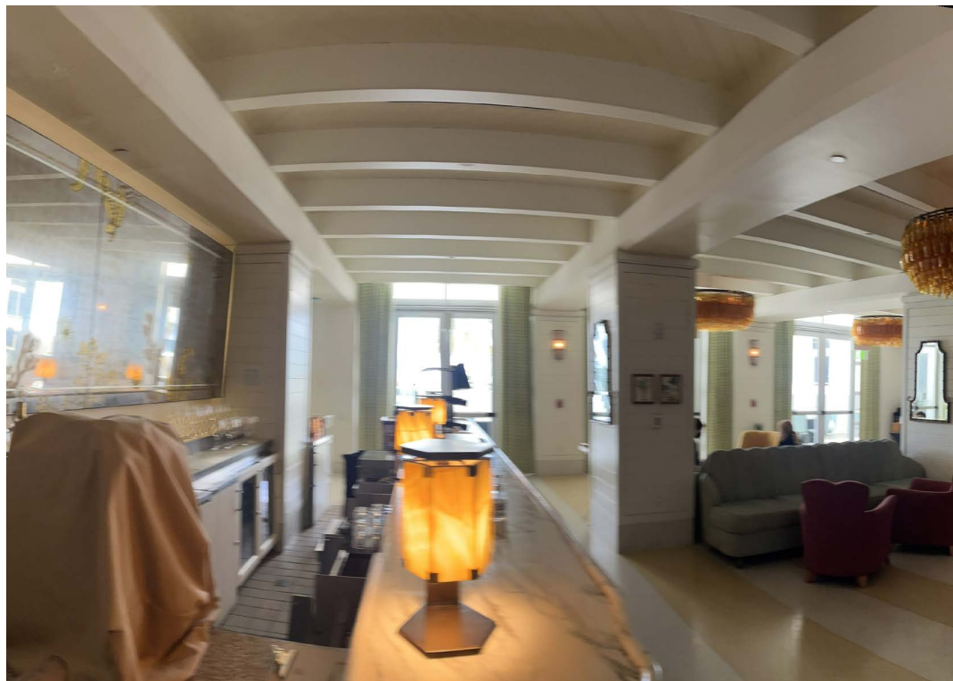
2ND FLOOR LOUNGE EXISTING CONDITIONS
