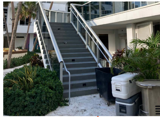
2ND FLOOR ACCESS
