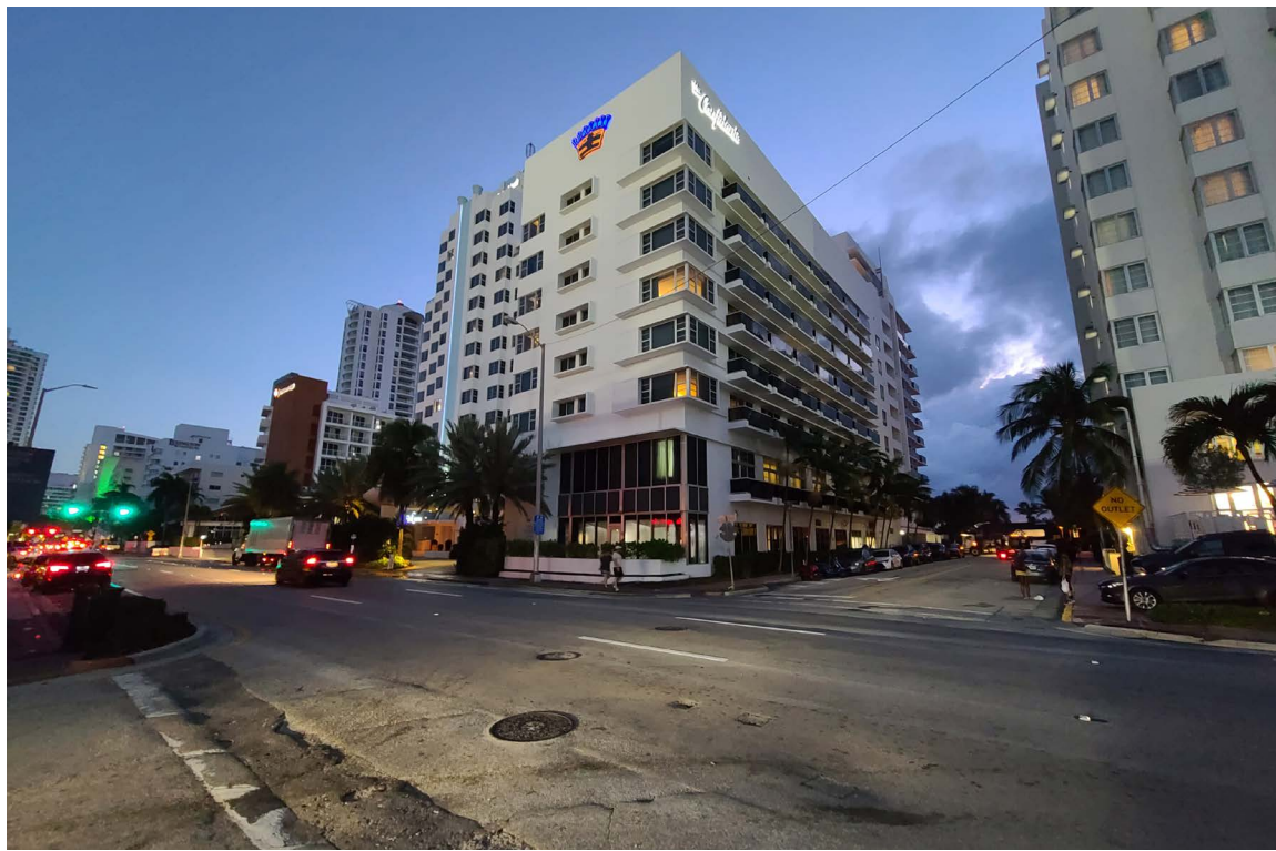
SOUTH WEST FACADE
