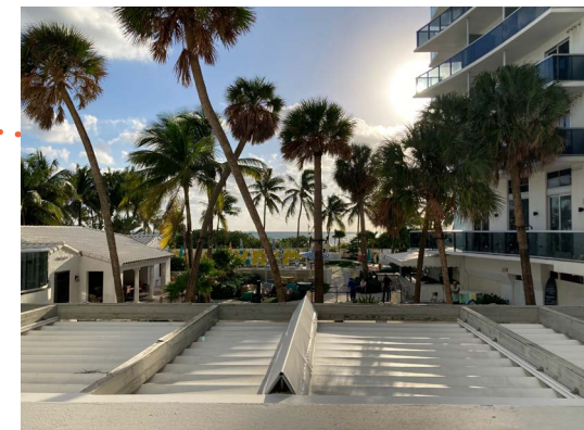
SECOND FLOOR CORRIDOR VIEW
