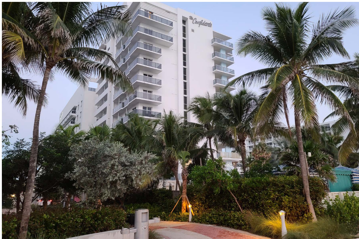
SOUTH EAST FACADE
