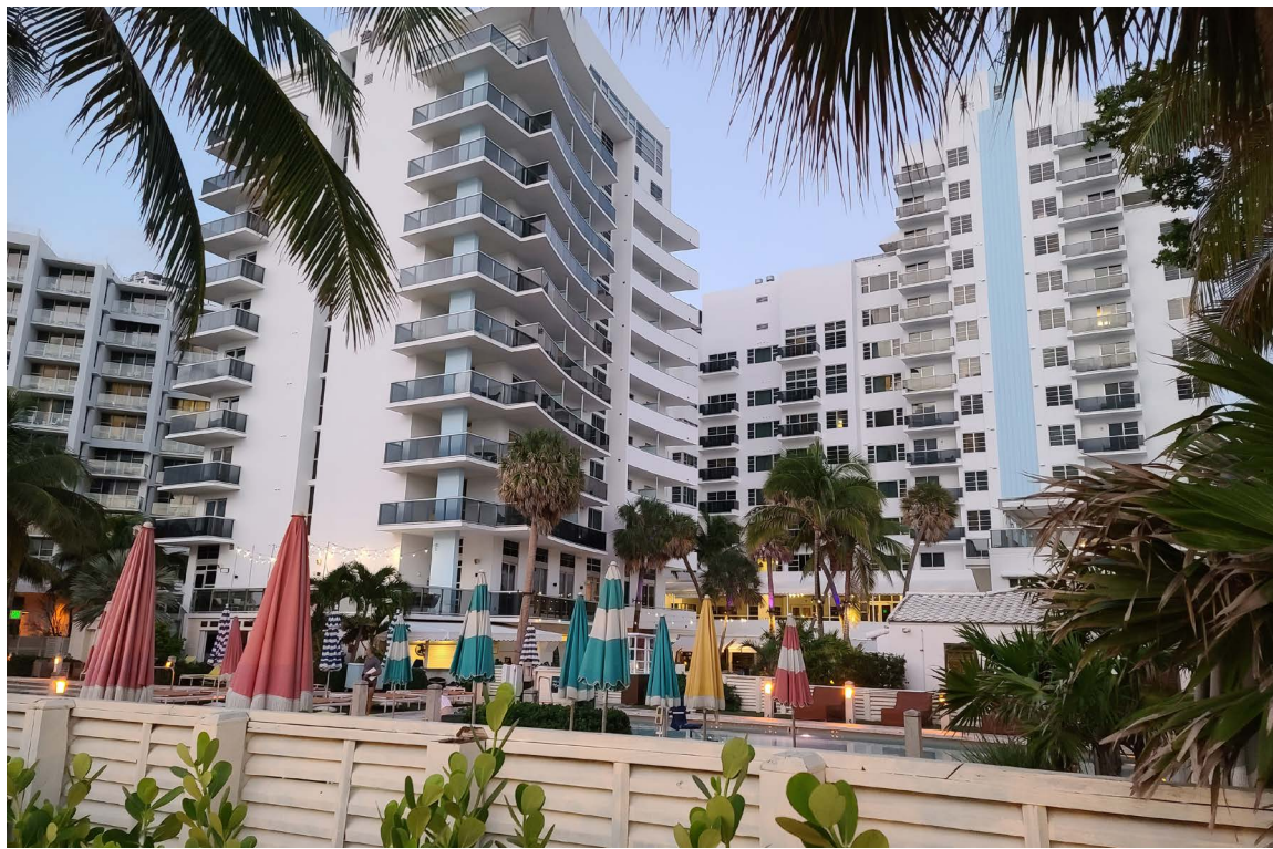
NORTH EAST FACADE
