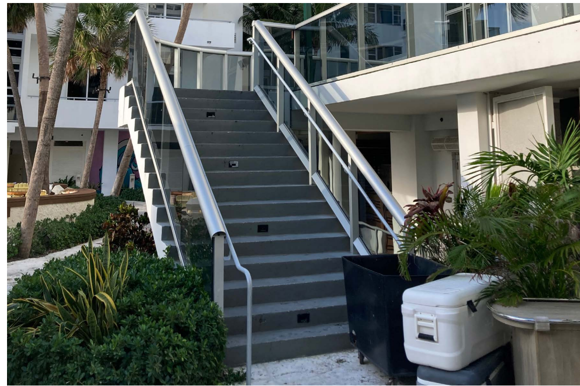
2ND FLOOR ACCESS
