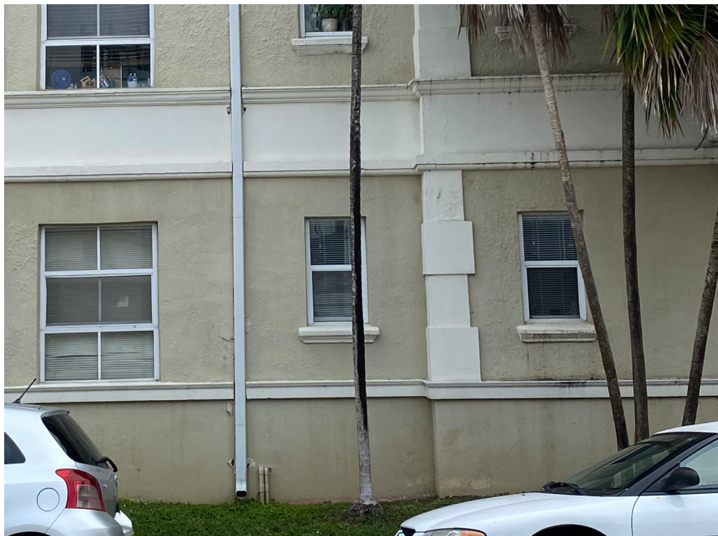
Park Avenue Facade - windows at ground level
