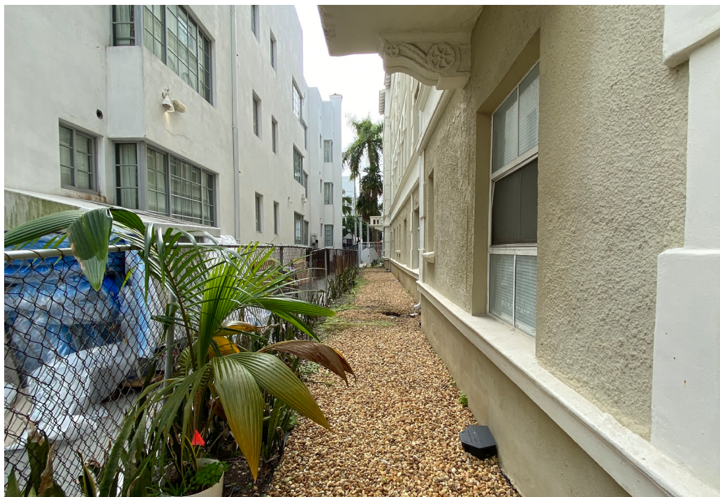
Looking South through West sideyard
