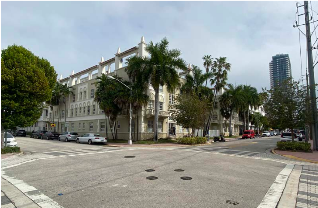
20th Street looking Northeast
