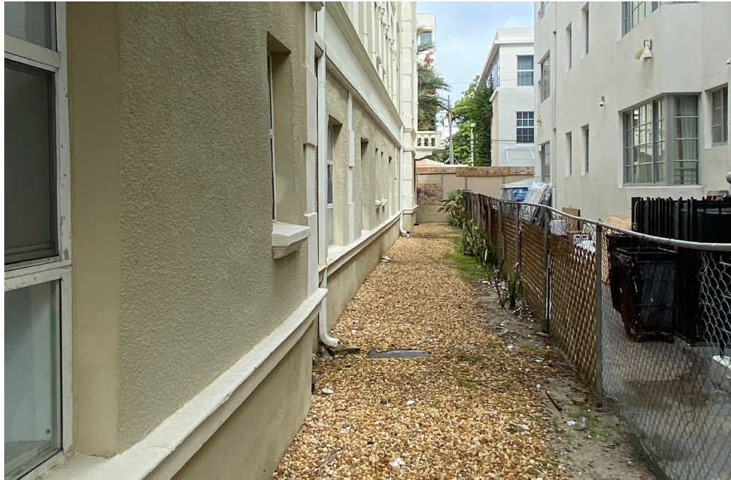
Looking North through West sideyard
