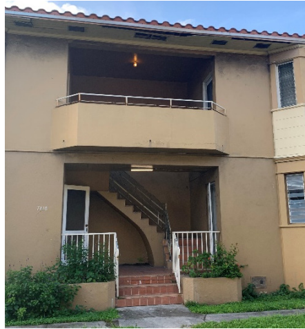
Fig. 34. Detail of outdoor staircases with inset balcony.
