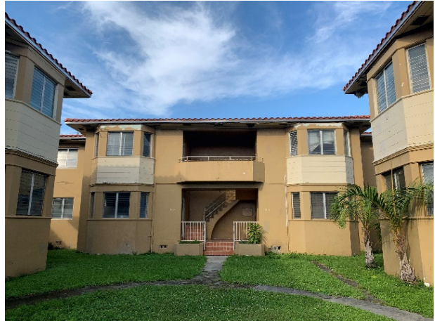
Fig. 32. East façade of West site building, January 2022.
