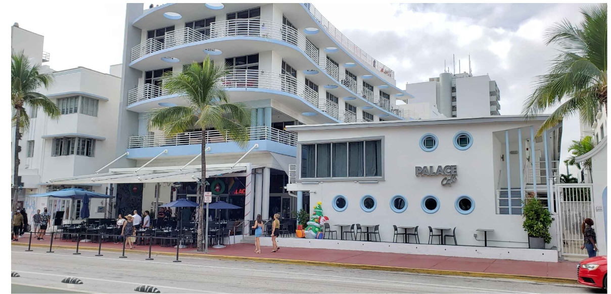
2. VIEW OF EXISTING SIDEWALK SEATING
