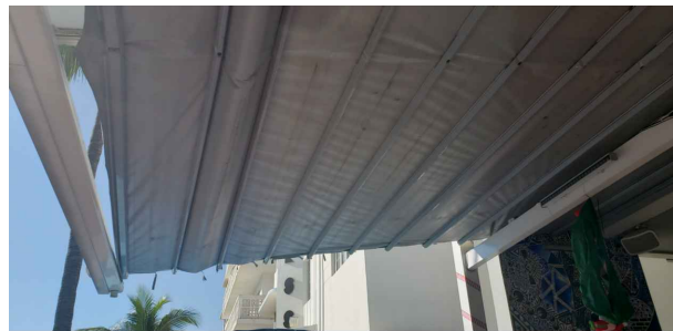
SUSPENDED CANOPY : OPAQUE PVC MATERIAL
