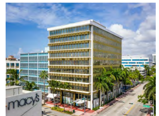
D MORRIS LAPIDUS 9 Story Commercial Building
