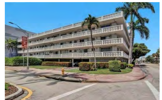
C JEFFERSONIAN CONDO 5 Story Residential Building
