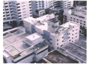
NORTH WEST VIEW
