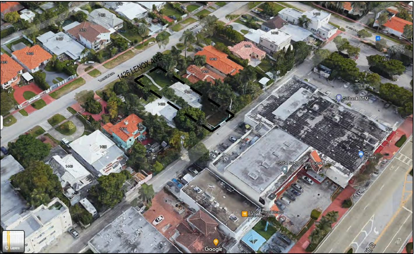
2 REAR AERIAL VIEW
