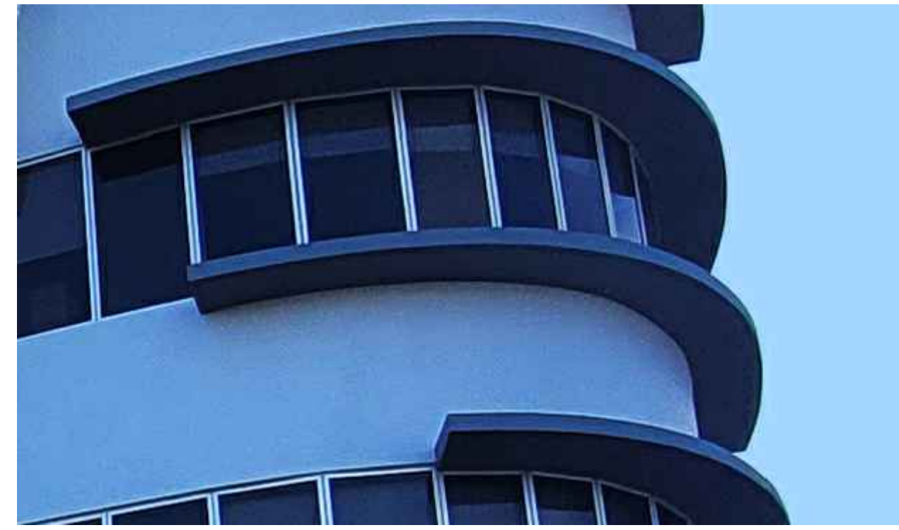
② EXISTING OFFICE BUILDING EYEBROW
