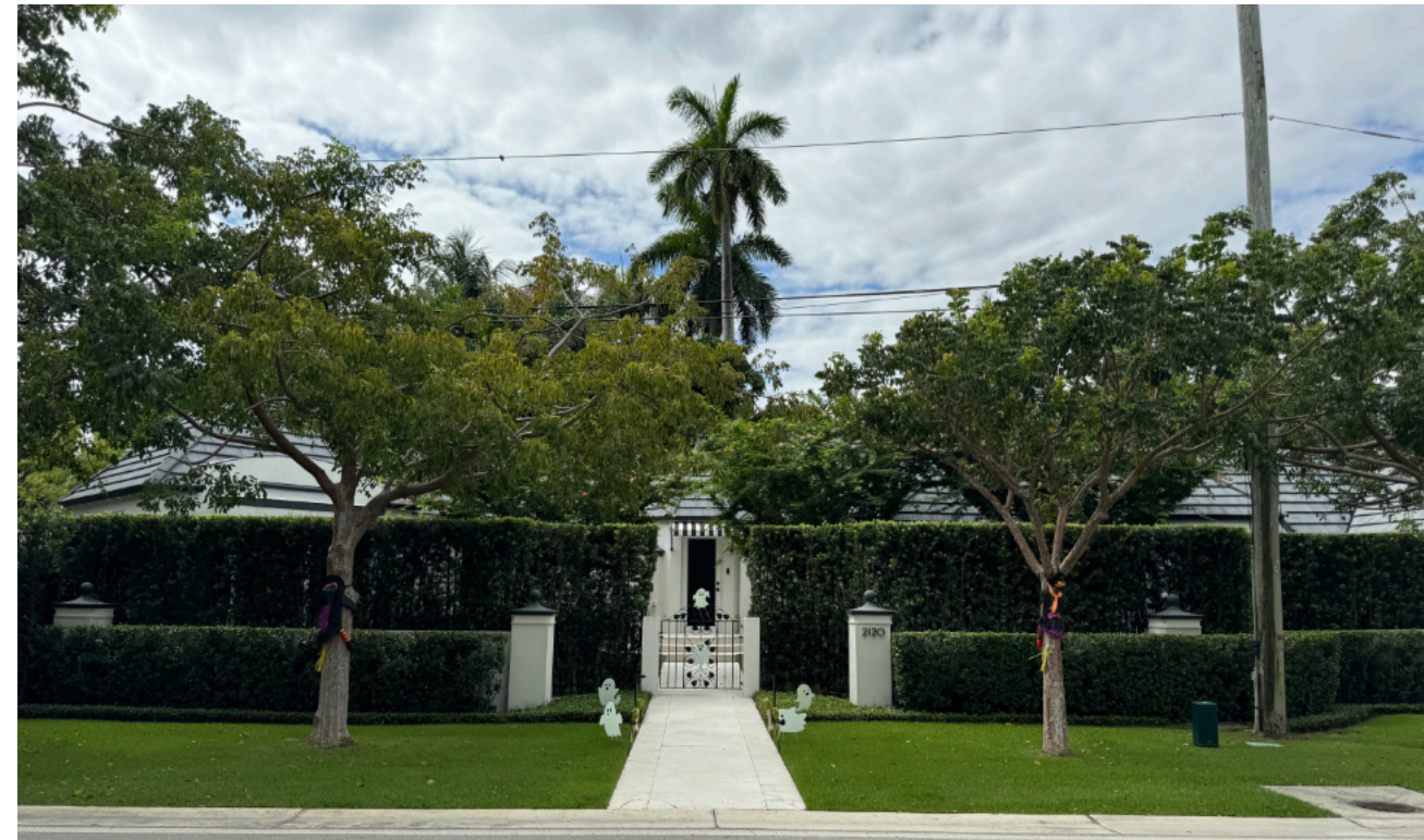
8 2120 SUNSET DRIVE EXISTING ONE-STORY RESIDENCE
