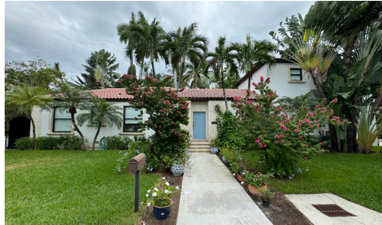
2 2111 REGATTA AVENUE EXISTING TWO-STORY RESIDENCE
