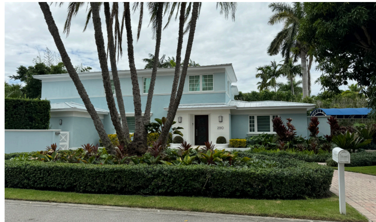
4 2130 REGATTA AVENUE EXISTING TWO-STORY RESIDENCE
