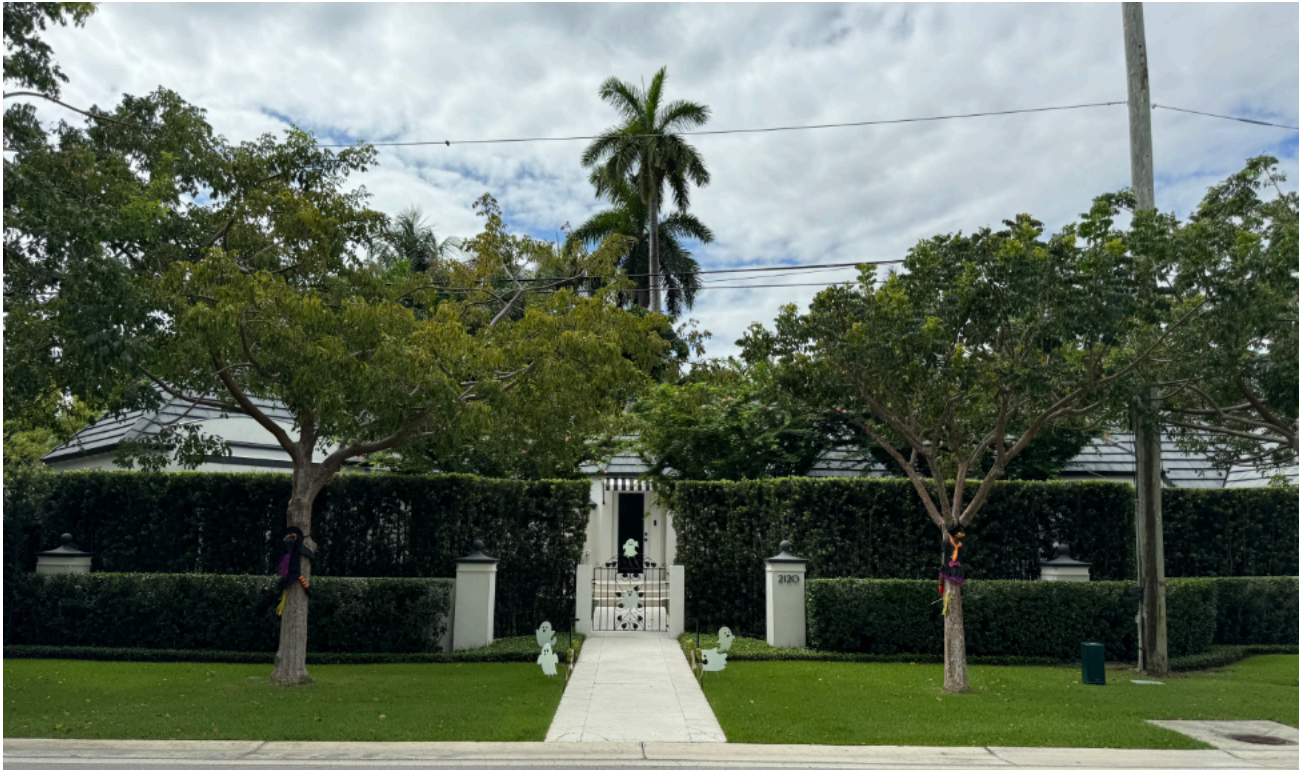
8 2120 SUNSET DRIVE EXISTING ONE-STORY RESIDENCE
