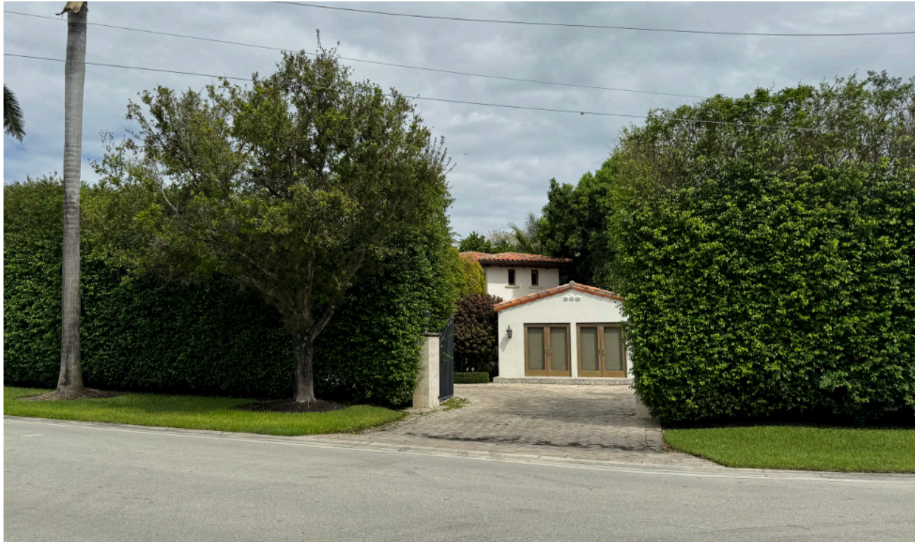
7 2201 SUNSET DRIVE EXISTING TWO-STORY RESIDENCE
