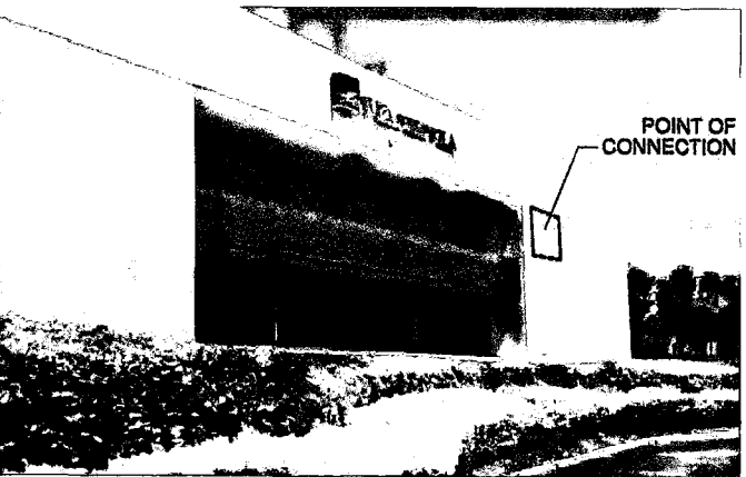
7 EXISTING SOUTH VIEW
