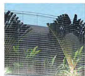
3 S.S. OR ALUMINUM SQUARE PENNING WIRE MESH PAINTED WHITE. 4" OPENINGS / NICKEL FINISH WIRE MESH
