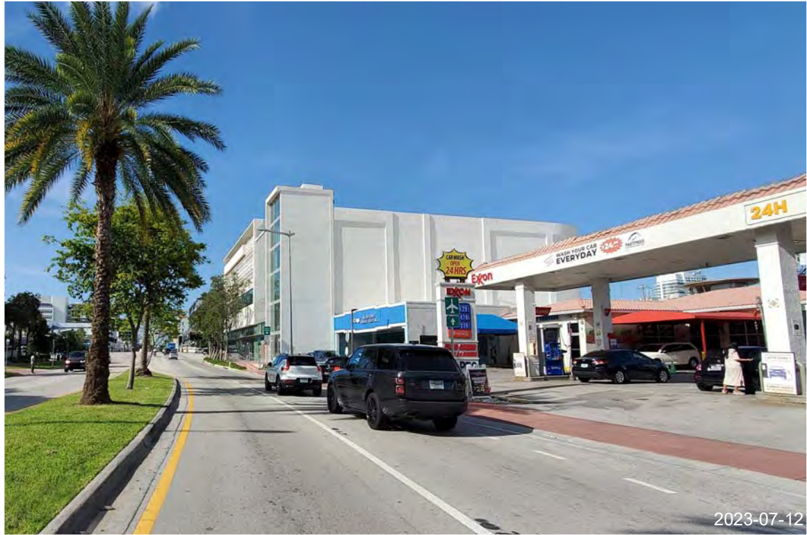
11. VIEW OF ALTON RD SOUTHWEST OF SITE
