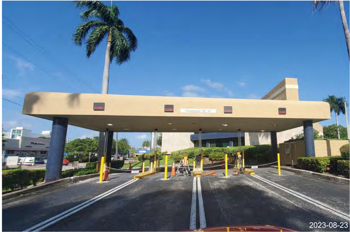
23.EXISTING DRIVE THRU BANK ON SITE
