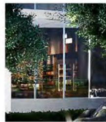
2 ALUMINUM-FRAMED STOREFRONT SYSTEM, W/ IMPCT-RESISTANT GLASS
