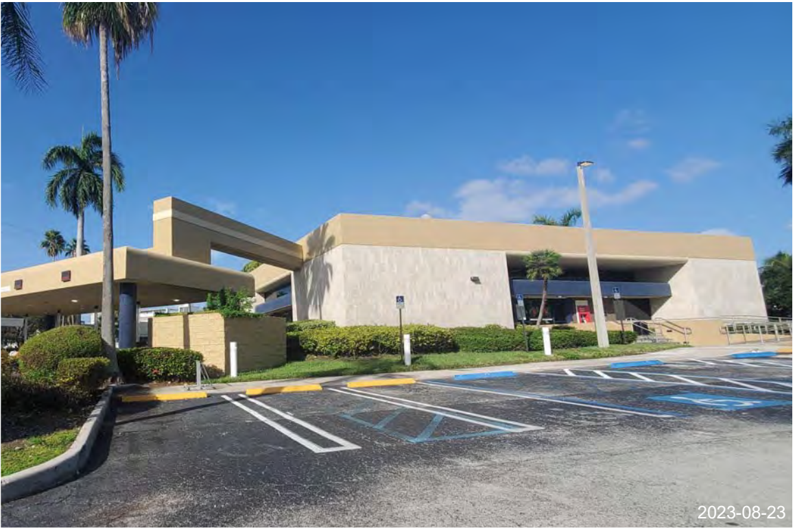
24. VIEW OF WELLS FARGO FROM EXISTING PARKING
