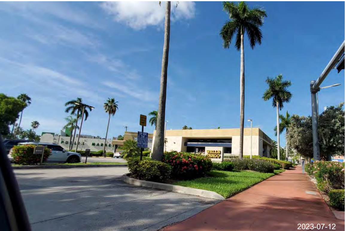
2. VIEW OF SITE FROM NORTH PEDESTRIAN WALKWAY
