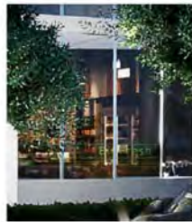
2 ALUMINUM-FRAMED STOREFRONT SYSTEM, W/ IMPCT-RESISTANT GLASS
