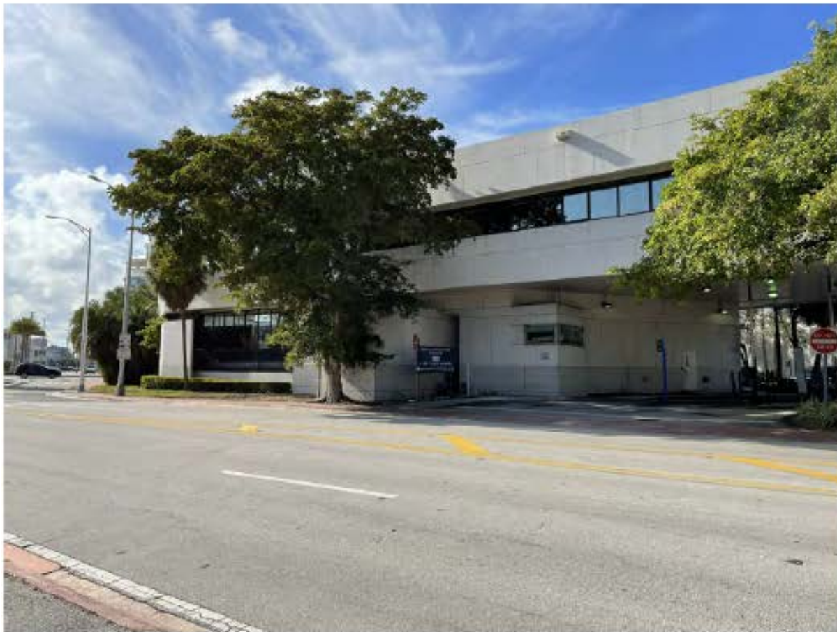
05 DADE BOULEVARD LOOKING NORTHWEST
