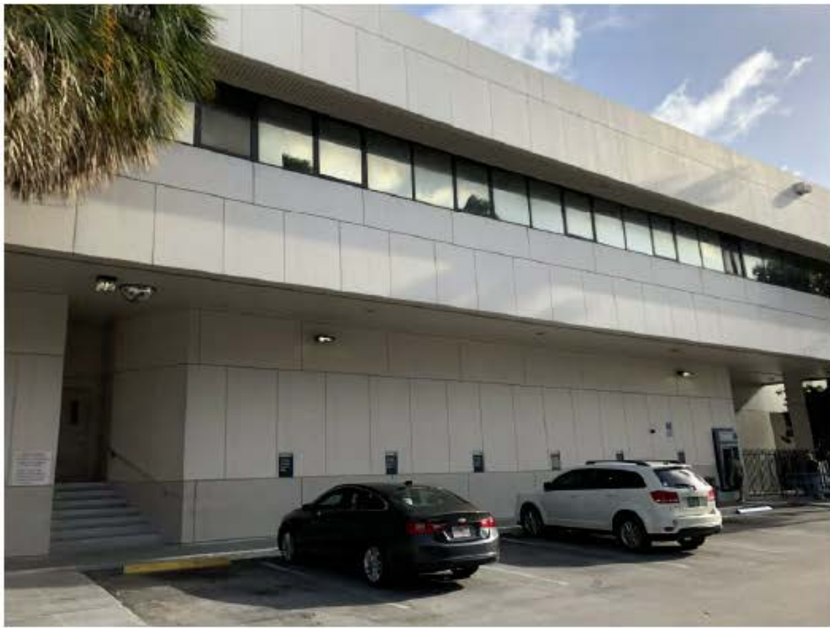
09 EXISTING PARKING LOOKING SW
