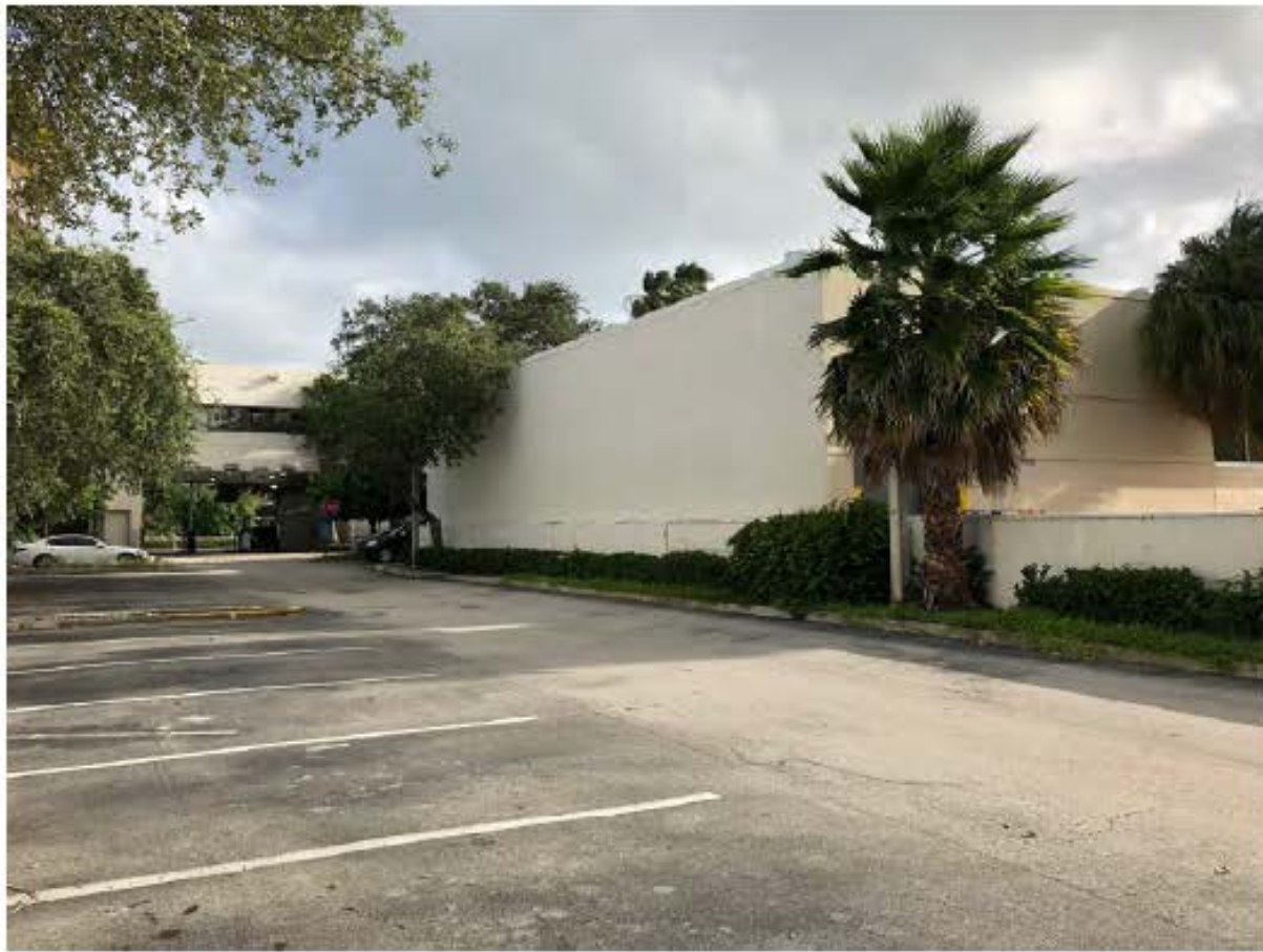
13 EXISTING PARKING LOOKING SW
