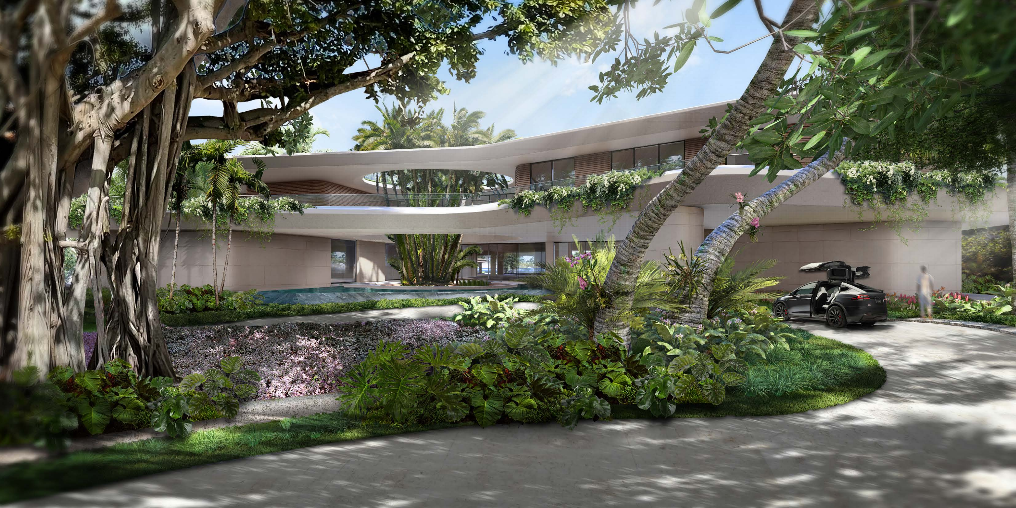
VIEW : MOTOR COURT
