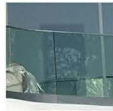
GL2 IMPACT GLASS HANDRAIL - CLEAR, RADIUSED CORNERS
