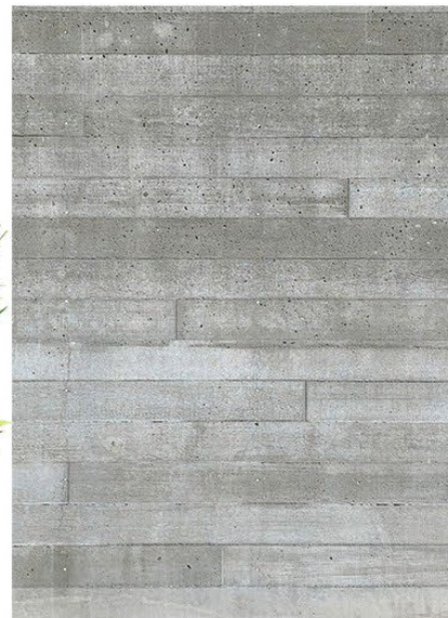
7. ARCHITECTURAL FEATURE WALL BOARD FORMED CONCRETE
