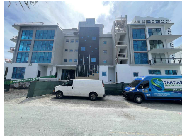
EAST NEIGHBOR CONSTRUCTION (8)
