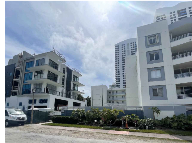
FRONT NEIGHBOR LOOKING EAST (6,7,8)
