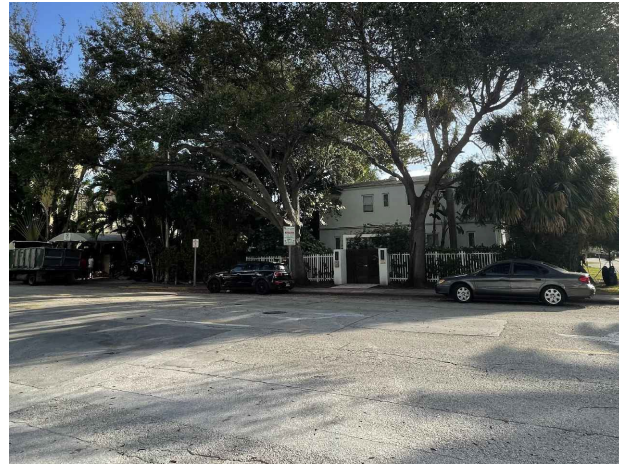
14TH TERRACE LOOKING EAST (9)
