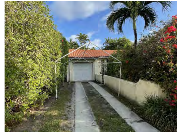
NEIGHBOR RIGHT SIDE NORTH (2)
