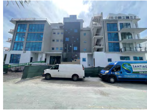
EAST NEIGHBOR CONSTRUCTION (8)
