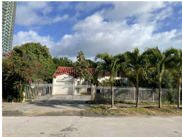
1339 14TH TERRACE EXISTING CONDITION
