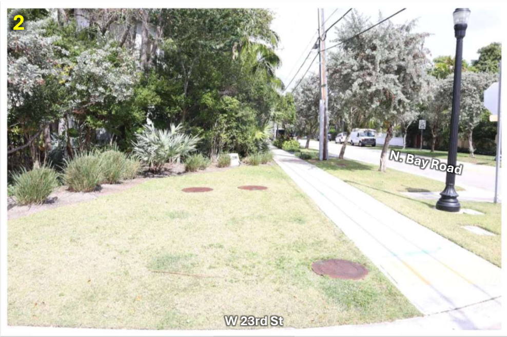
Existing Stormwater Utilities Looking North Along W 23 rd Street
