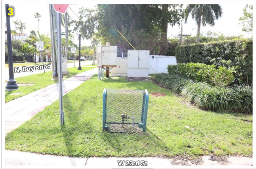
Existing Communication & Water Utilities Looking South Along W 23 rd Street
