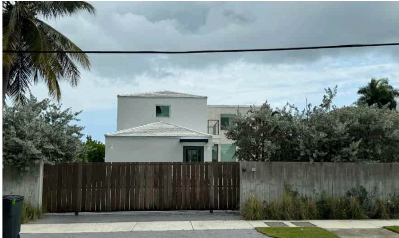
5 403 E. DI LIDO DRIVE EXISTING TWO-STORY RESIDENCE
