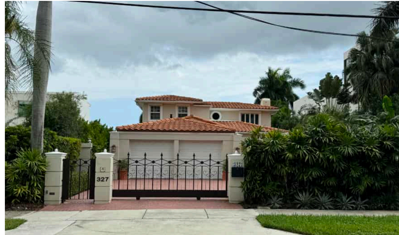
6 327 E. DI LIDO DRIVE EXISTING TWO-STORY RESIDENCE
