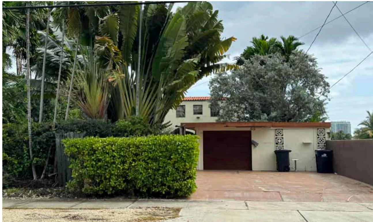
3 415 E. DI LIDO DRIVE EXISTING TWO-STORY RESIDENCE
