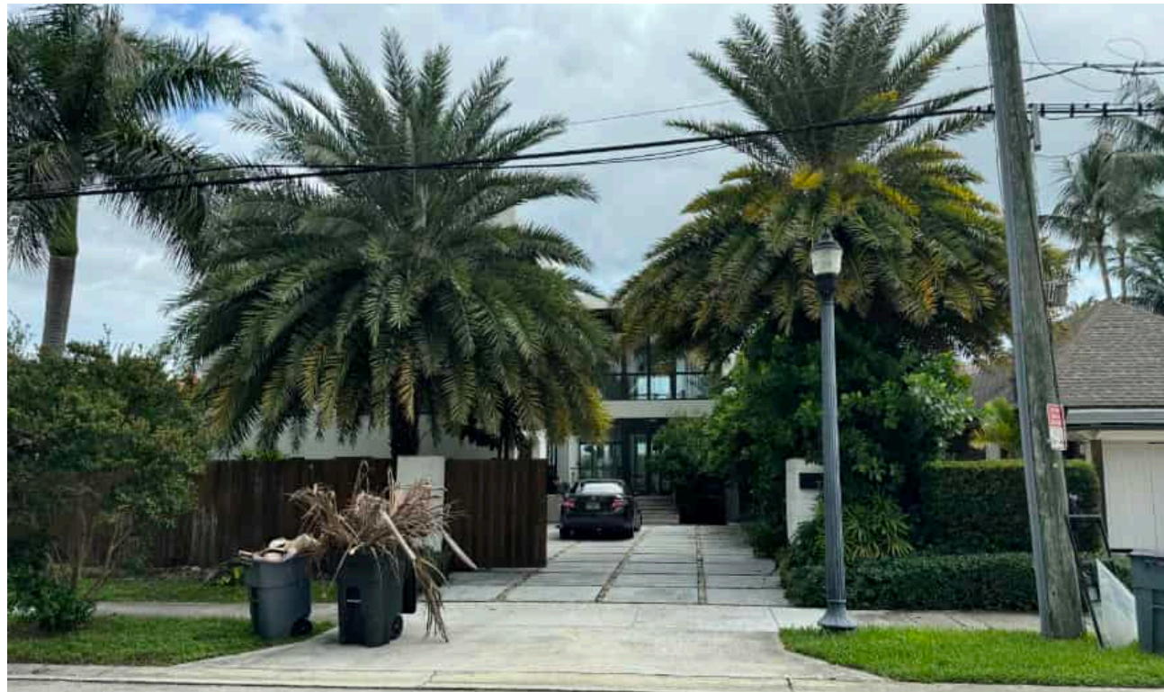
7 321 E. DI LIDO DRIVE EXISTING TWO-STORY RESIDENCE
