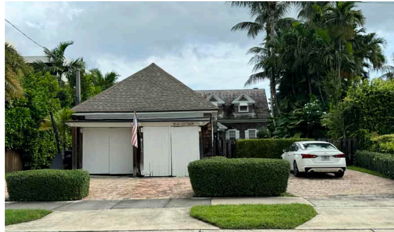
8 315 E. DI LIDO DRIVE EXISTING TWO-STORY RESIDENCE
