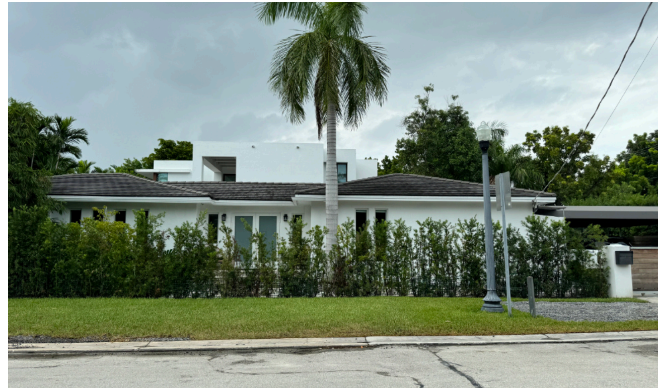
12 424 E. DI LIDO DRIVE NEW ONE-STORY RESIDENCE
